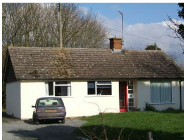
Woolaway bungalow with precast concrete panels
