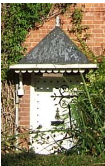
Pretty lead canopy over painted timber door
