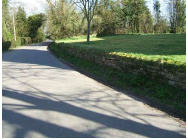
Low dry stone wall boundary around the church yard
