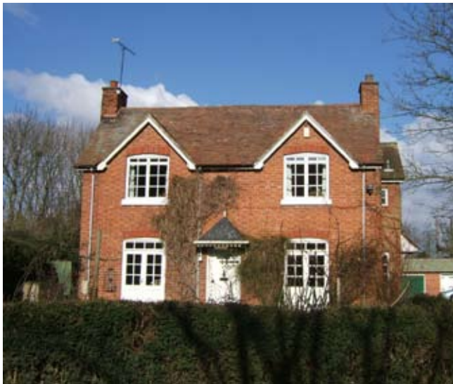
Houses typically have more complex plan, are two storey with painted timber casements arranged symmetrically
