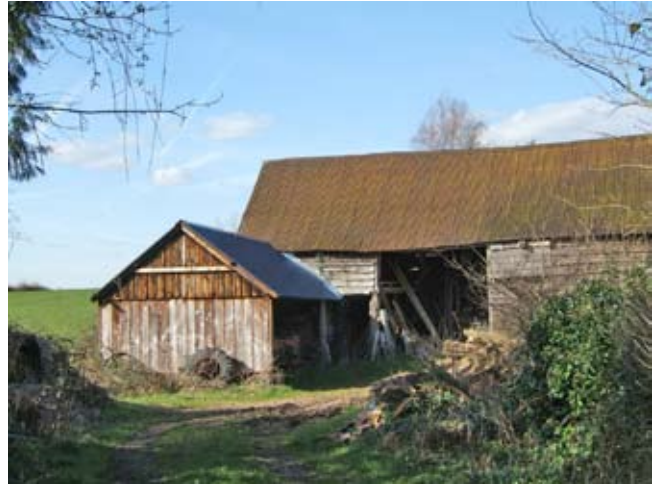
Nibbles barn is timber framed - this was common in the midlands during the 16 th and 17 th centuries
