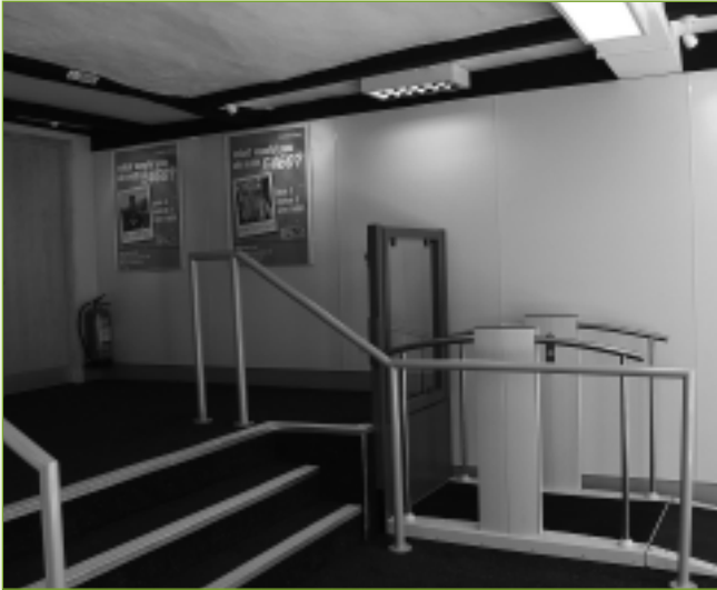
Platform lifts are less obtrusive than a long ramp with hand rails - High Street Pershore
