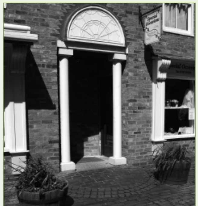
This ramp is a practical & attractive solution to making easy access over the step - High Street Pershore
