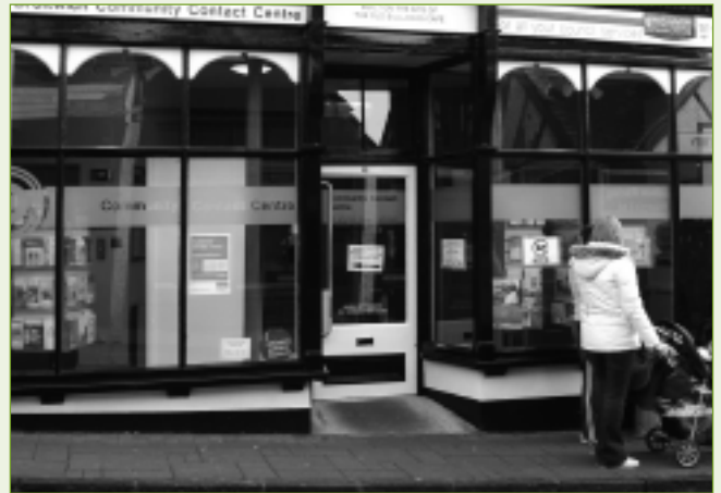
Droitwich Contact Centre has a ramp to allow access over the step.
