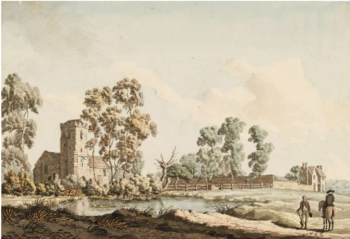
Figure 21: Picture (circa 1780's) of Church and Hampton Court beyond viewed from the west - showing its rural setting
