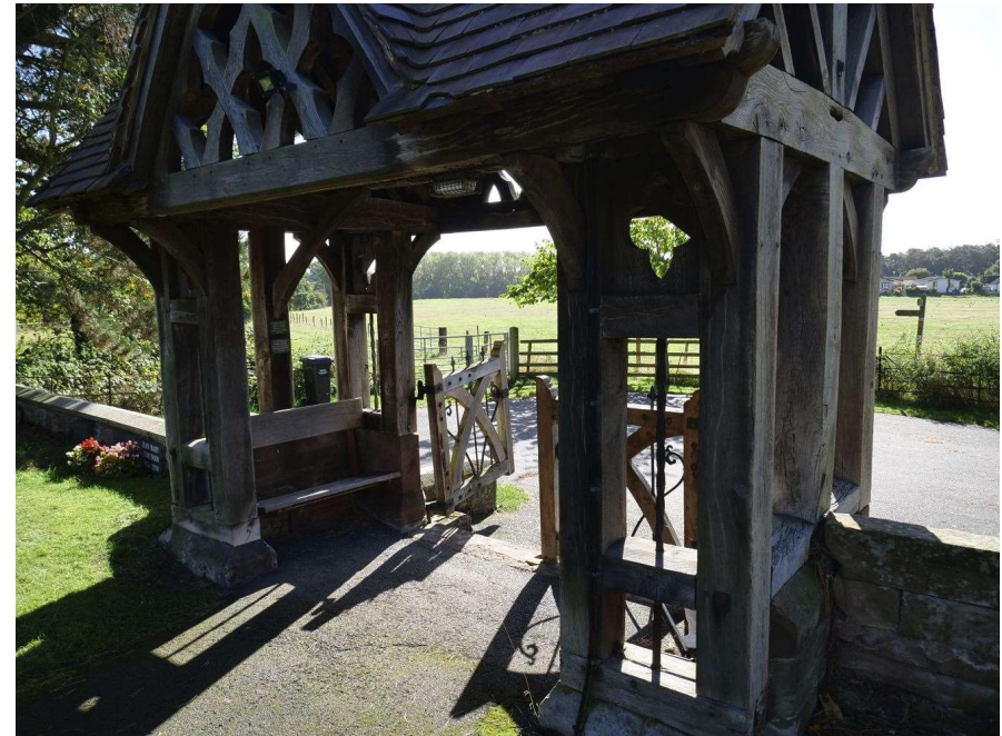
Figure 11: View of the Lych-gate structure and architectural detailing
