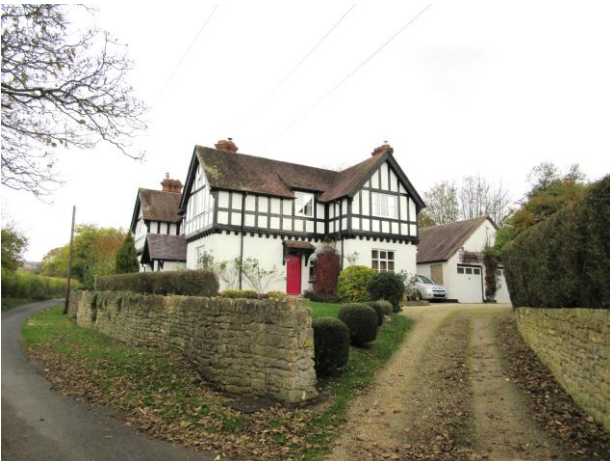
19th century Lodge Cottages make use of traditional materials but in a design characteristic of its period of construction
