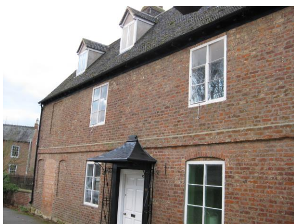
Dalton House with its casement windows. The ground floor windows show cambered brick heads.
