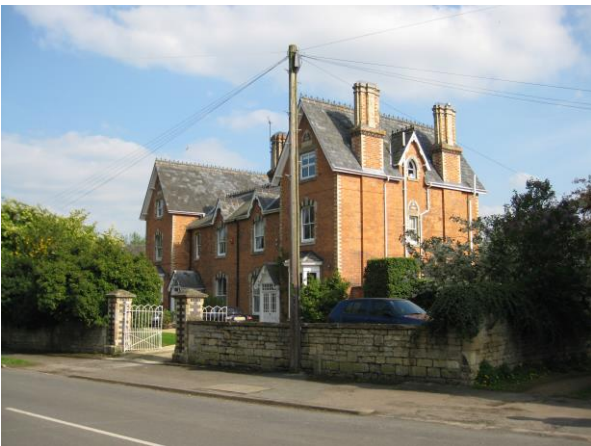
19 th century semi detached properties, steep roof pitches with two matching chimneys in roof elevation at either end
