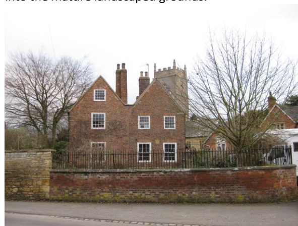
The low stone boundary wall with its railings permitting views into the garden area.
