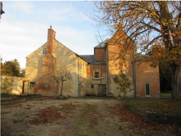
The west elevation of The Old Vicarage, the mixed use of materials becomes more prominent here
