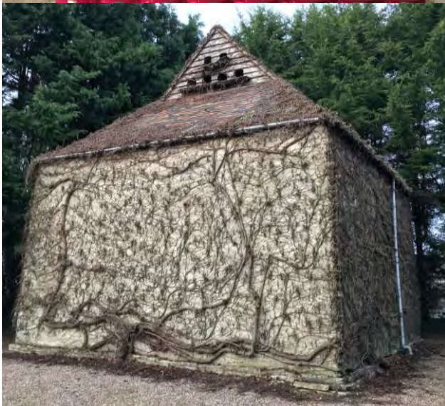
The exterior and interior of the converted Theatrebarn, and the Dovecote to the rear of the barn
