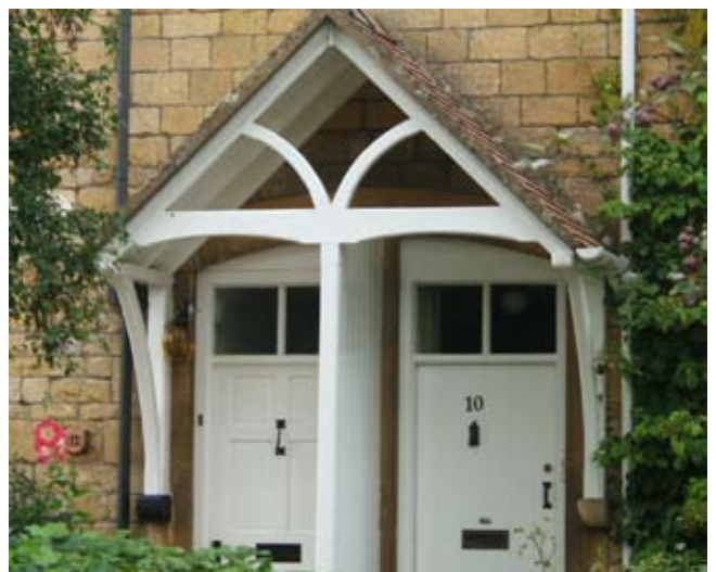
Some cottages have modest but well detailed open timber porches
