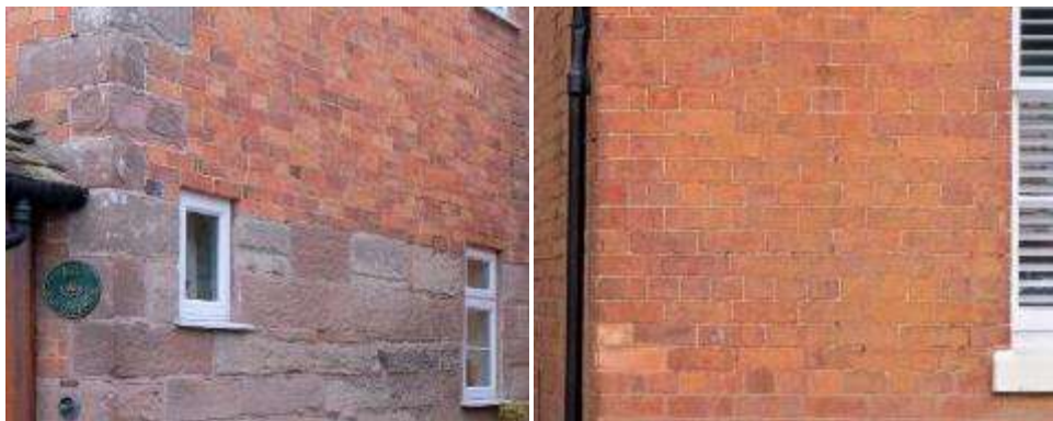
A hybrid brick and stone wall in Inkberrow (left) and a wall with fine pointing in Ombersley (right)
