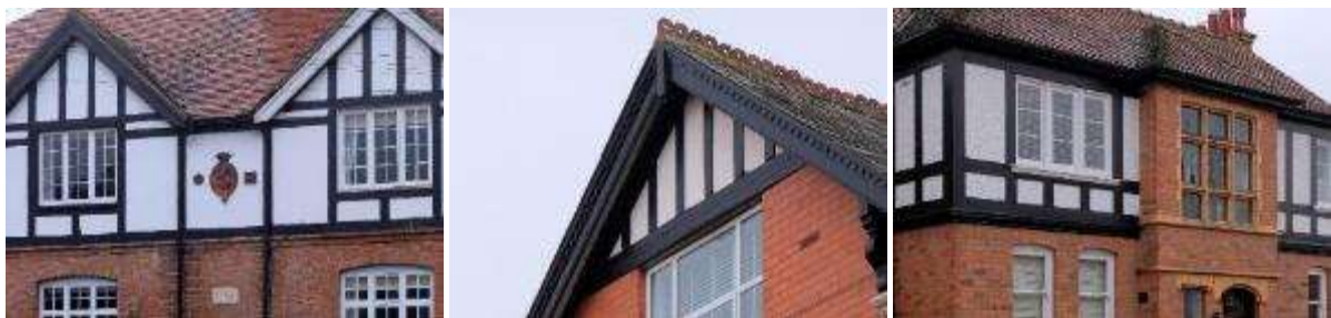
Late Victorian and Edwardian timber framing was usually not structural but ornamental, such as these examples in combination with brick walls in Inkberrow (left) and in Droitwich Spa (centre and right)
