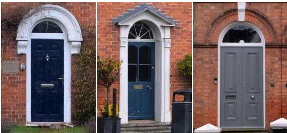
Doors with semi-circular fanlights and classical detailing in Inkberrow (left and centre) and Droitwich Spa (right)
