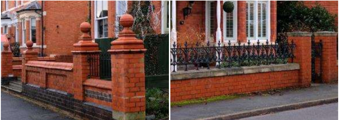
In Droitwich Spa, highly ornamented brick walls with brick banding and finials (left) and a brick wall with cast iron railings (right)
