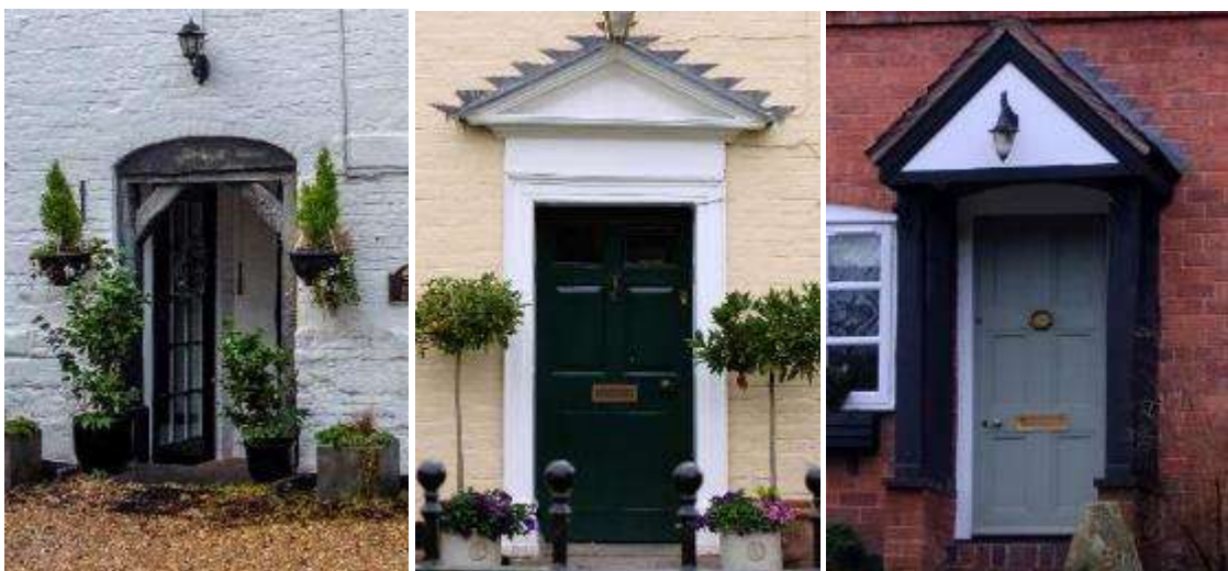
A recessed glazed door in Inkberrow (left), a Georgian-style door with pediment in Ombersley (centre) and a narrow porch in Uphampton (right)
