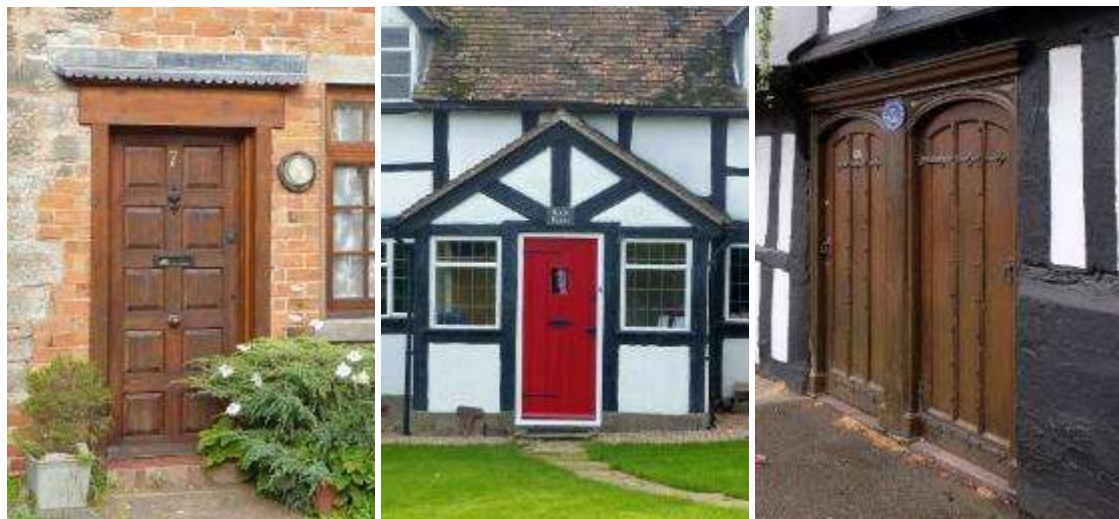
In Inkberrow, timber panelled doors in a vernacular style with a simple overhang (left) and within an enclosed porch (centre) and double doors in Ombersley (right)
