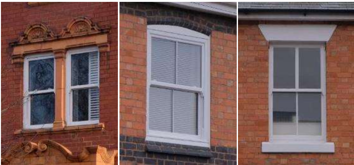
1-over-1 (left) and 2-over-2 (centre and right) sash windows in Droitwich Spa
