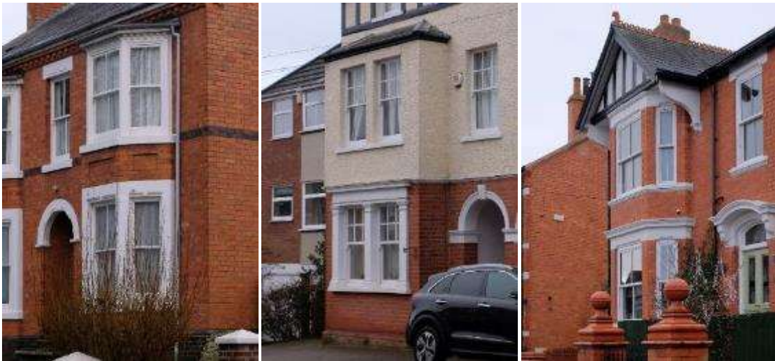
In Droitwich Spa, two-storey bay windows with contrasting white and brick (left), with a rendered first storey (centre) and with a prominent timber-frame gable (right)
