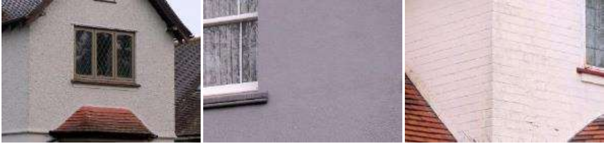
Roughcast (left), lilac render (centre) and painted brick (right) in Droitwich Spa
