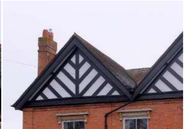
Timber frame detailing can be added to brick buildings, but these should not appear as "stuck on" elements. Where this is used, eaves should be at least 200mm deep.
