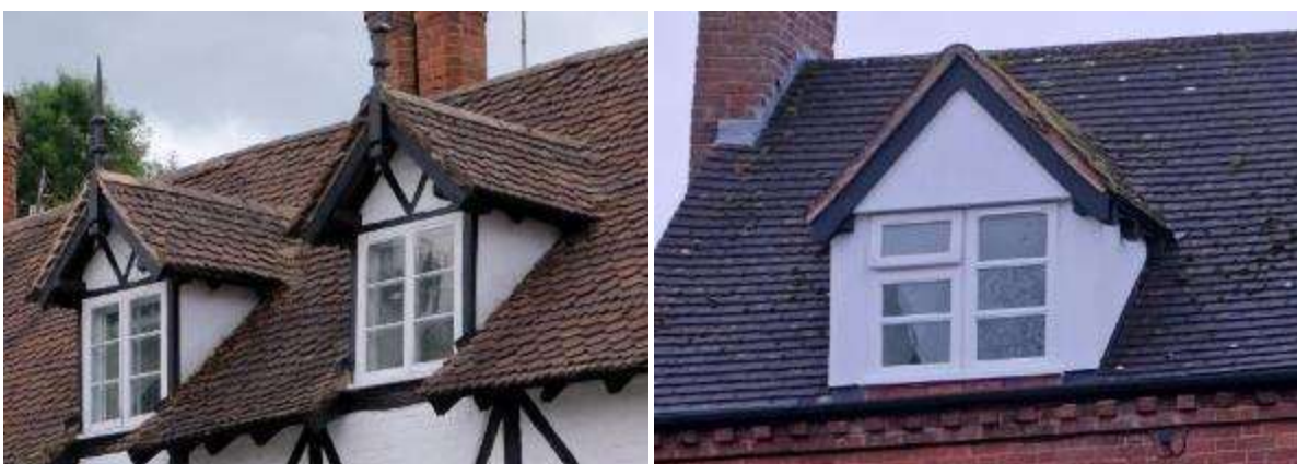
Timber-framed dormer windows in Ombersley (left) and a wide simple dormer in Uphampton (right)
