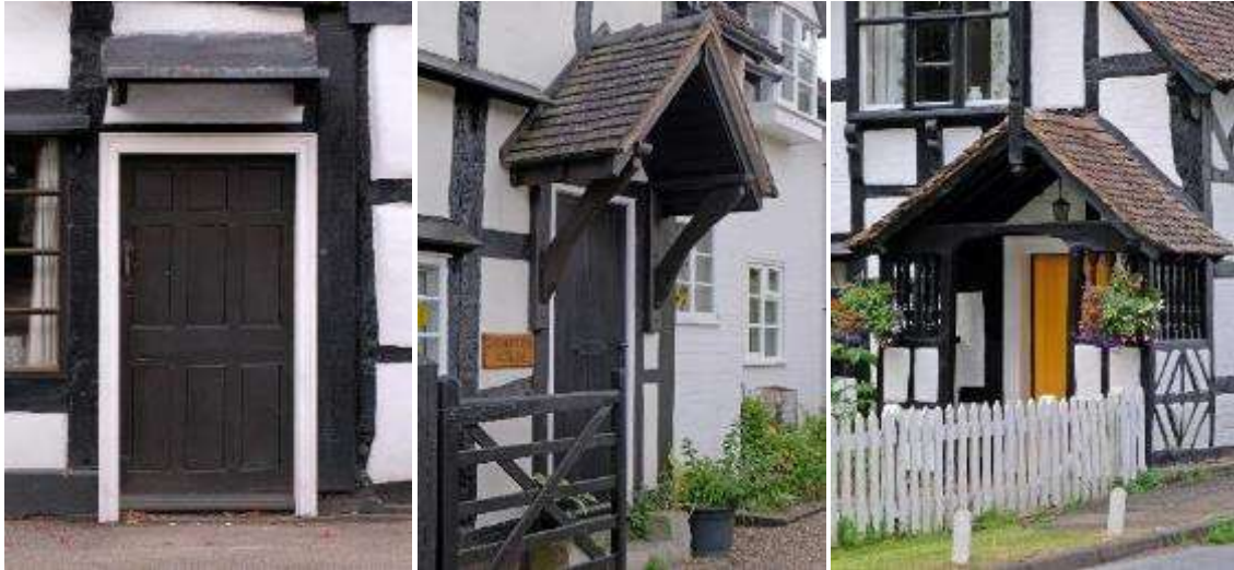
Timber panelled doors in a vernacular style in Ombersley and with a variety of door canopies and a large porch
