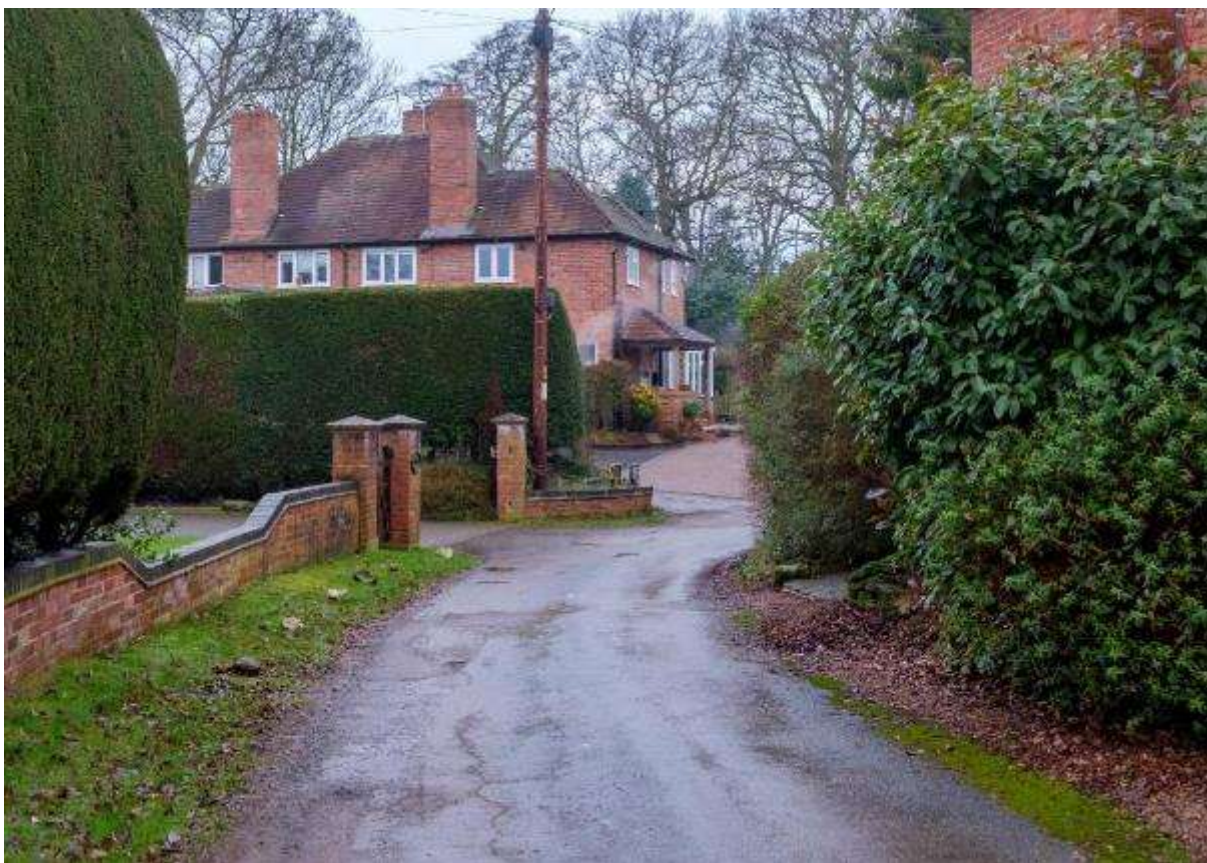
On streets without kerbs, such as this street in Uphampton, verges can play an important role in absorbing rain runoff without the need for extensive infrastructure
