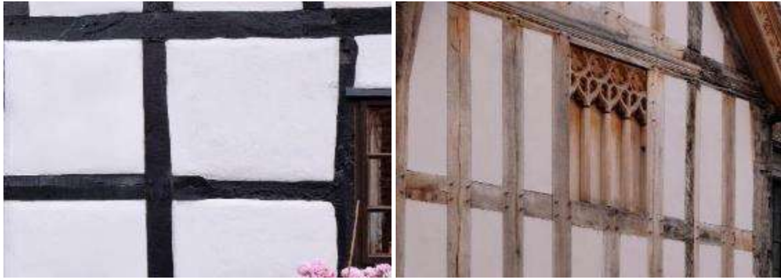
Timber framing in Ombersley with a smooth render infill (left) and an unpainted timber frame in Droitwich Spa (right)
