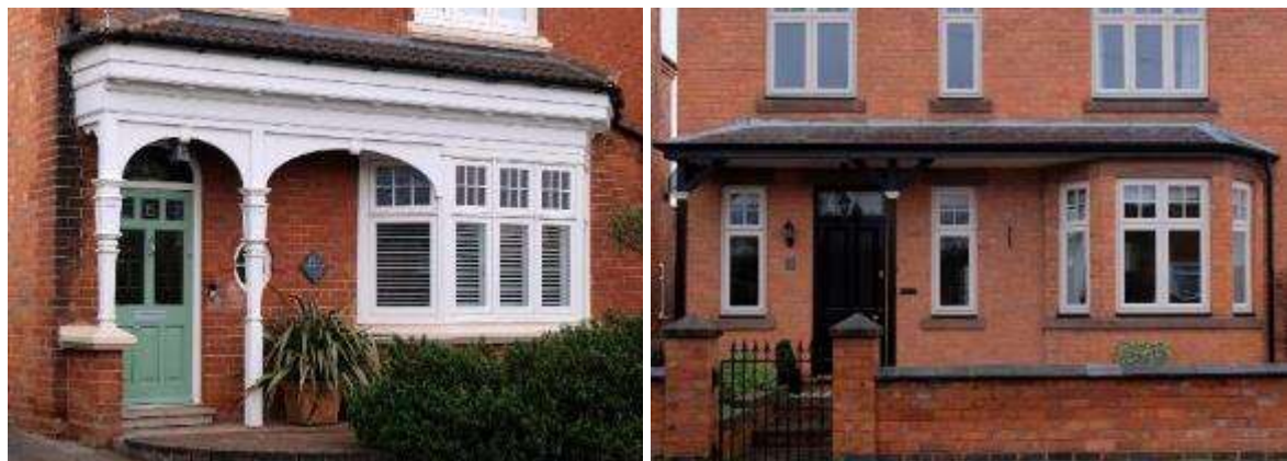
Combination door canopies and bay windows in Droitwich Spa with white trim (left) and in brick (right)
