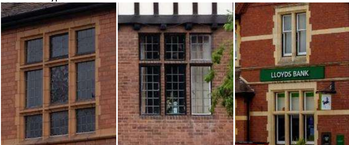
In Droitwich Spa, fixed leaded windows (left), leaded windows with brick transom and mullions (centre) and with stone transom and mullions (right)
