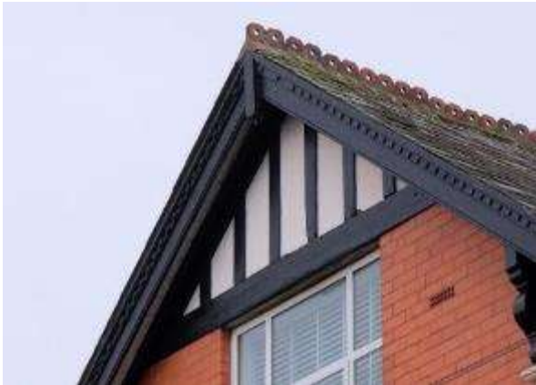
Timber frame detailing can be added to brick buildings, but these should not appear as "stuck on" elements. Where this is used, eaves should be at least 200mm deep.
