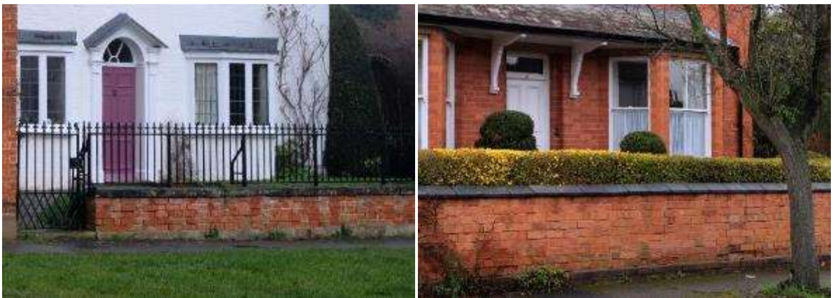
A brick wall with delicate cast iron railings in Inkberrow (left) and a brick wall with black coping bricks and a hedge above in Droitwich Spa (right)
