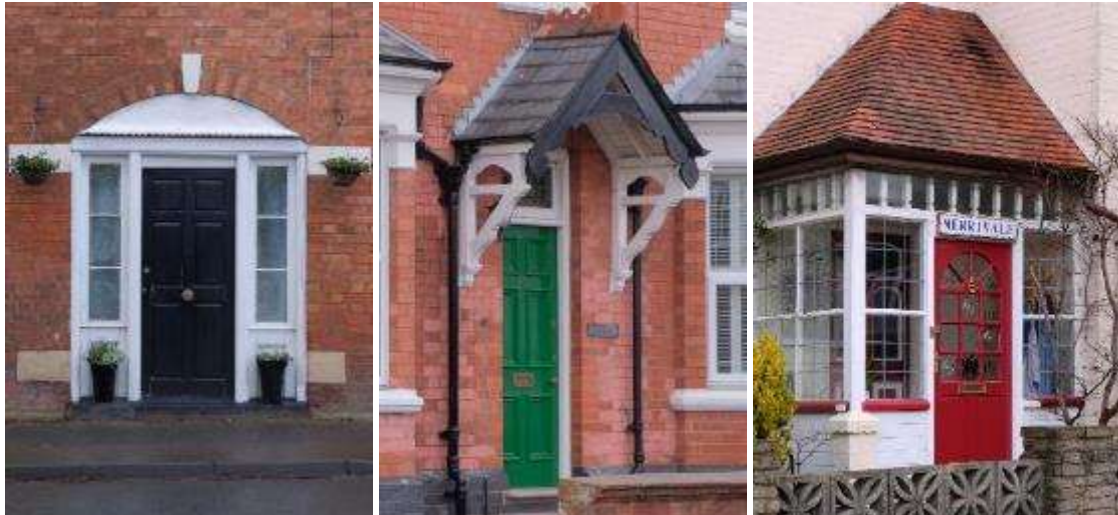
A door in Inkberrow with windows either side (left) and in Droitwich Spa doors with ornamented canopies (centre) and an enclosed porch (right)
