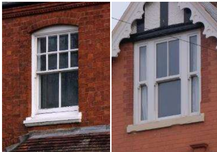
8-over-2 windows (left) and combo sash windows (right) in Droitwich Spa
