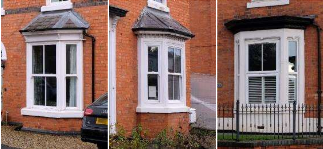
In Droitwich Spa, bay windows with pitched roofs and corbels (left and centre) and a simpler bay window with a prominent cornice (right)
