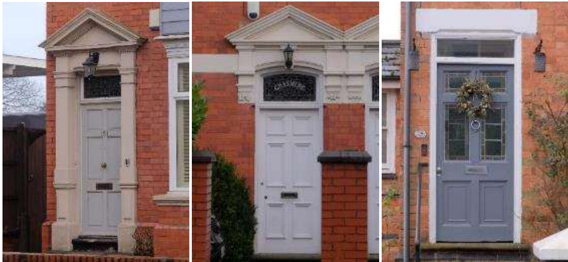
Doors in Droitwich Spa with classical pediments and transom lights
