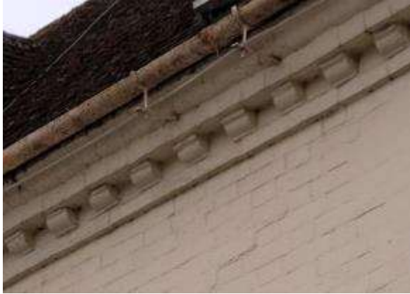
In Droitwich Spa, a dentil cornice (left) and a highly ornated example (right)
