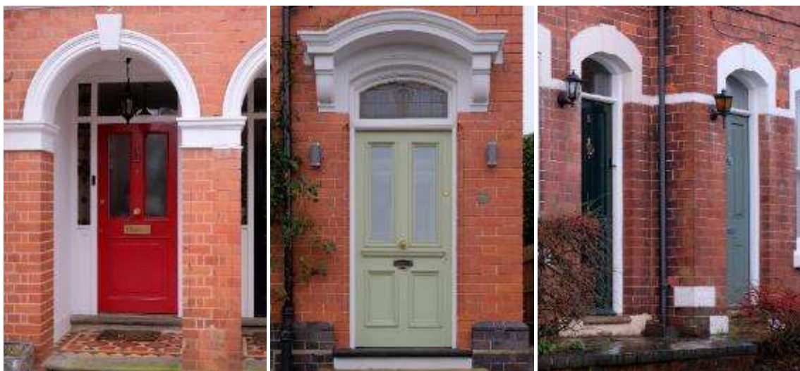
In Droitwich Spa, a recessed door surrounded by glazing (left) and a door with an arched canopy (centre) and two doors with arched transom lights in Hartlebury (right)
