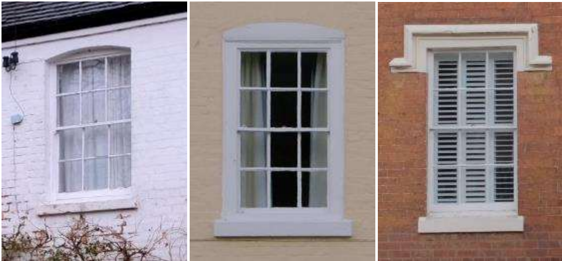
6-over-6 sash windows in Uphampton (left) and Ombersley (centre and right)
