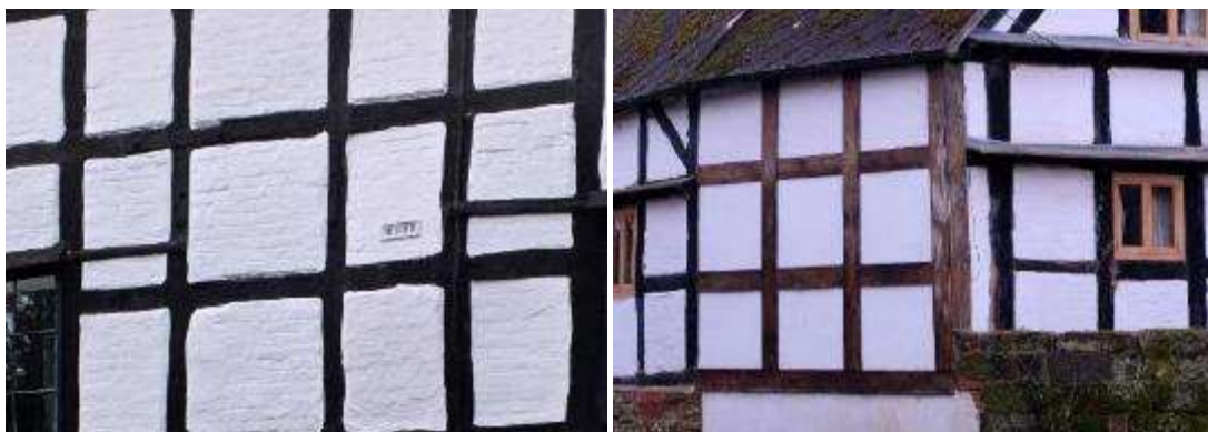
Timber framing with painted brick nogging in Inkberrow (left) and both painted and unpainted in Uphampton (right)
