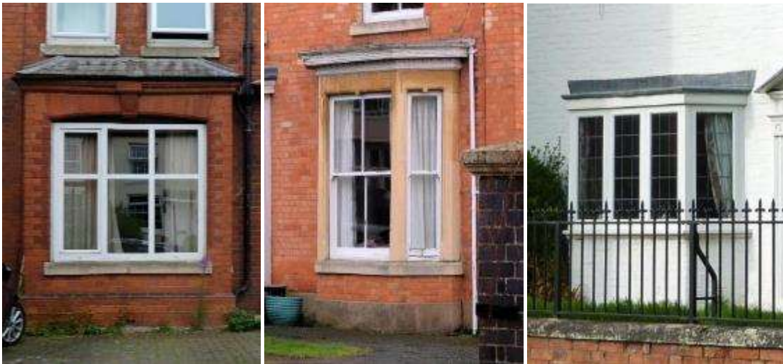
In Droitwich Spa (left and centre), a brick box bay window and a brick and stone bay window, and in Inkberrow (right) a simple all-white bay window
