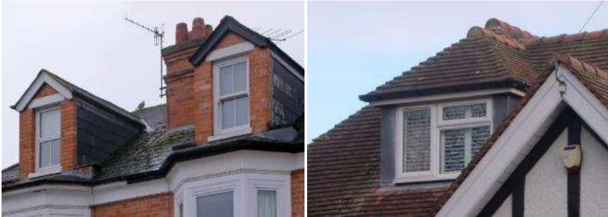
Brick dormer windows (left) and a single large dormer with hipped roof (right) in Droitwich Spa
