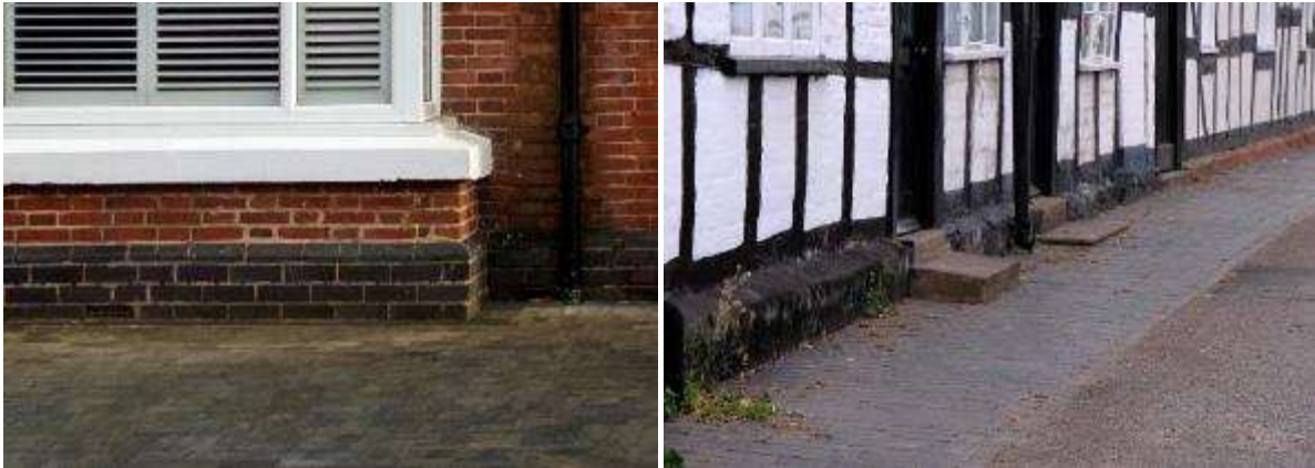
A burnt brick plinth in Droitwich Spa (left) and painted and unpainted stone plinths in Ombersley (right)
