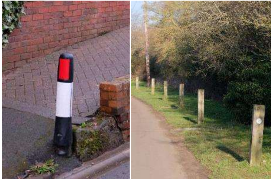
Plastic bollards such as this one in Hartlebury (left) must not be used. Instead, in villages and rural areas, timber bollards are a more sympathetic option, such as these in South Littleton (right)
