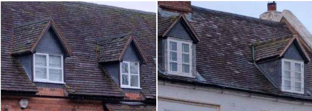
Pairs of pitched-roof dormer windows with lead flashing in Uphampton (left) and Hartlebury (right)
