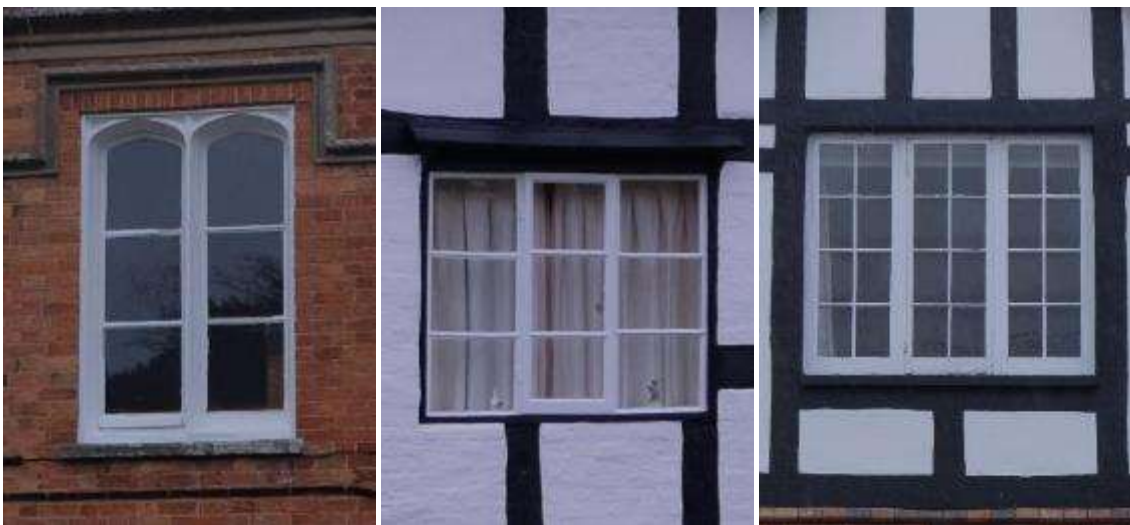
3 pane arched windows in Inkberrow (left), fixed panes with a central casement in Uphampton (centre) and 8 pane windows in Inkberrow (right)
