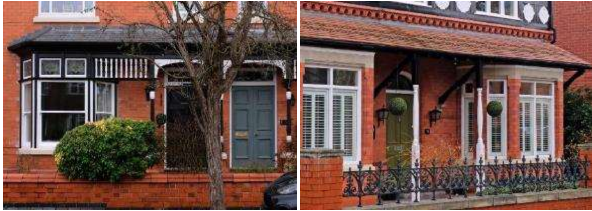
Door canopies spanning between bay windows in Droitwich Spa
