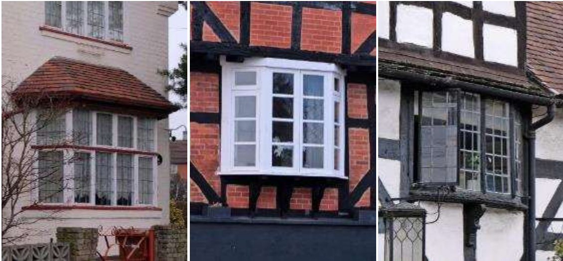
A large Arts & Crafts style bay window in Droitwich Spa (left) and delicate oriel windows supported by corbels in Hartlebury (centre) and Ombersley (right)
