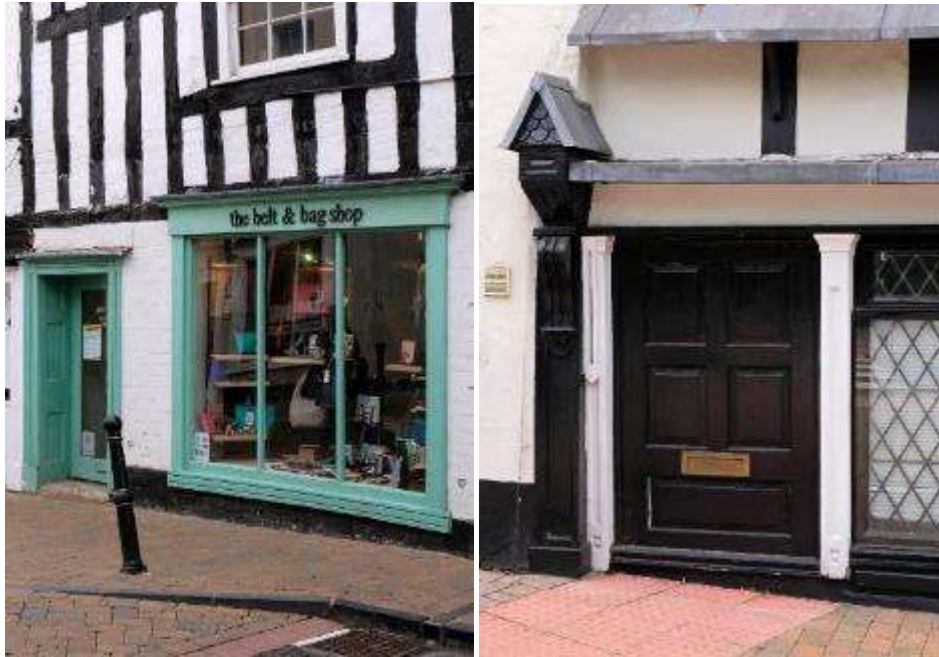
Shopfronts in Droitwich Spa with locally characteristic detailing
