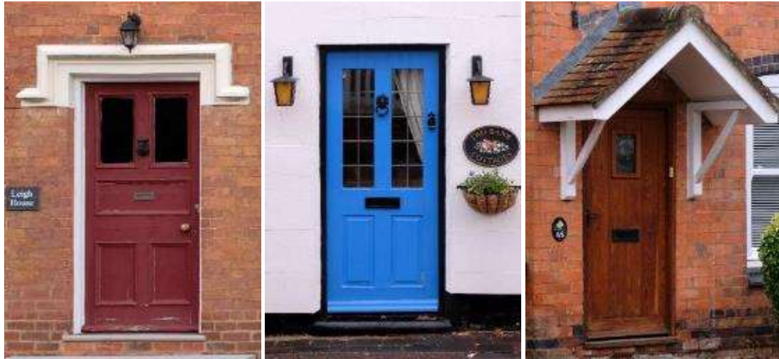
Doors with glazing and a variety of panel patterns, and with a hood mould in Ombersley (left), with two lanterns either side in Hartlebury (centre) and with a large canopy in Droitwich Spa (right)
