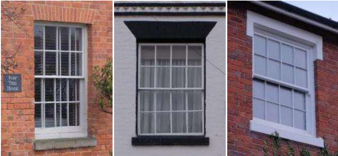
8-over-8 sash windows with a variety of lintel types in Inkberrow (left), Ombersley (centre) and Hartlebury (right)
