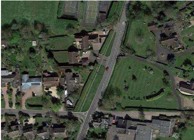
In Inkberrow, a verge distances a footpath from the busy road
