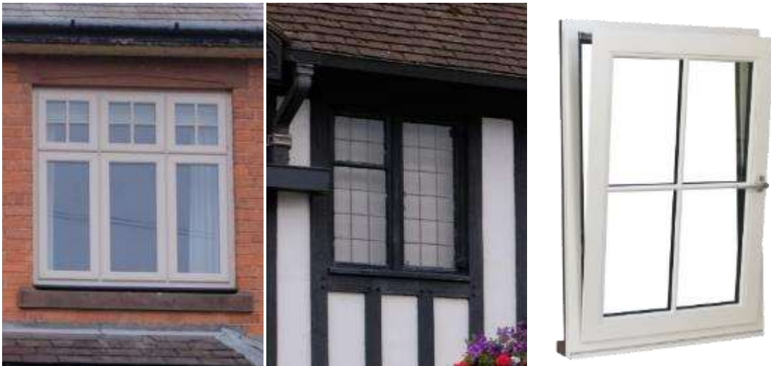
In Droitwich Spa, casements with top hung panels and transoms and mullions (left and centre) and a modern inward opening tilt/turn timber window (right, image credit George Barnsdale)
