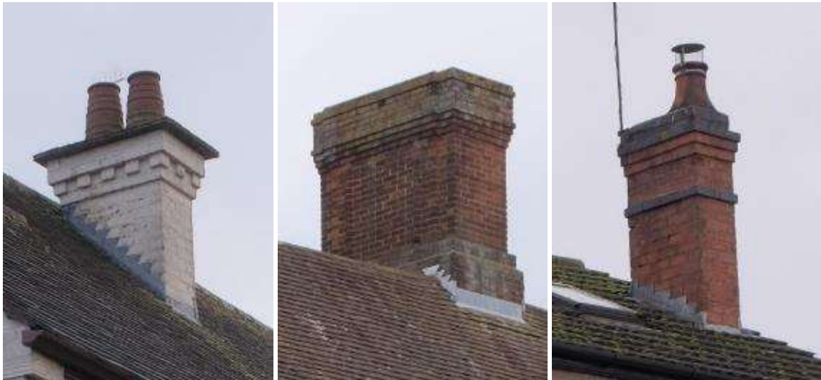
In Droitwich Spa, a painted brick chimney with dentils (left) a large chimney with corbels (centre) and a smaller example with corbels (right)
