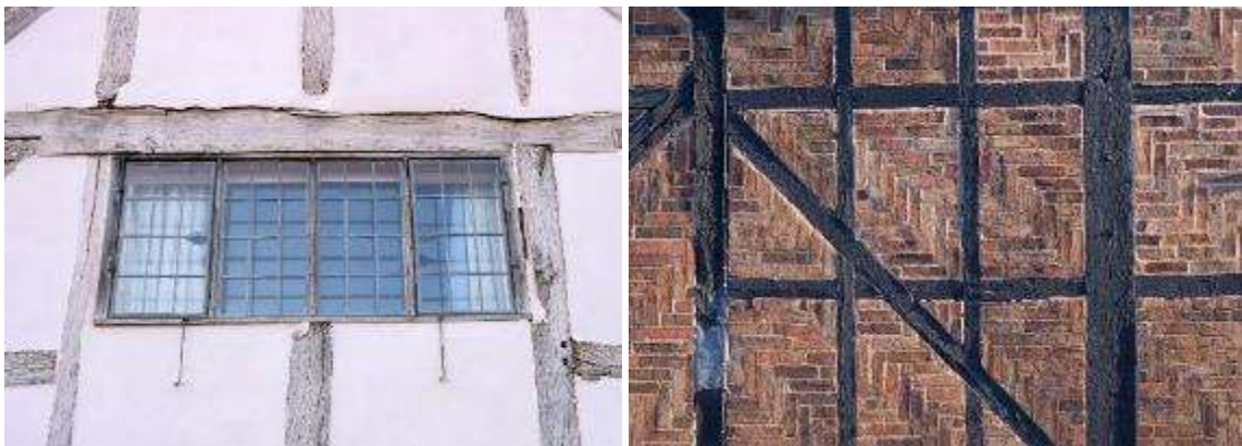
An unpainted timber frame and unpainted brick nogging in Norton
