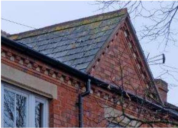
In Evesham, dentilled eaves corbels (left) and an elaborate brick frieze (right)
