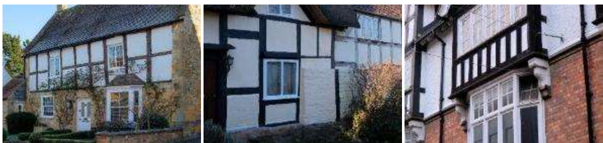
Hybrid timber frame homes alongside stone walls in Honeybourne (left), Norton (centre) and with brick and render in Evesham (right)
