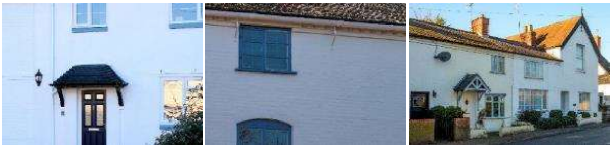
Painted brick in Harvington (left), Pebworth (centre) and South Littleton (right)
