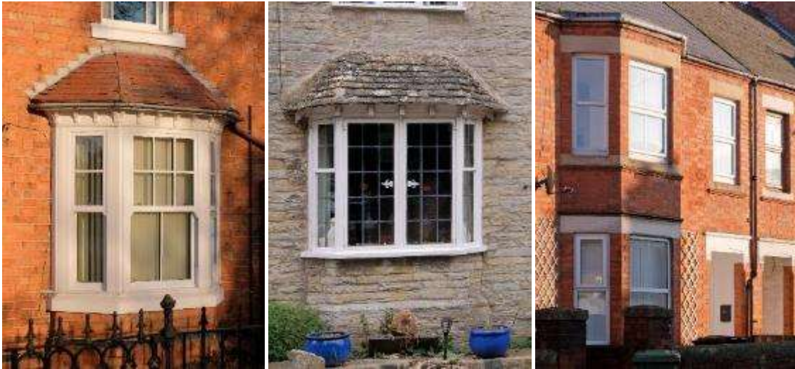
Bay windows with pitched roofs and dentils in Harvington (left) and Cleeve Prior (centre) and a two storey bay window in Evesham (right)
