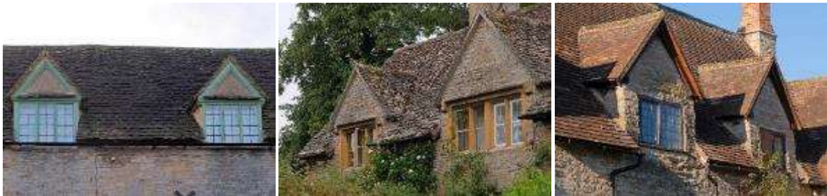
Pairs of dormer windows on lias stone houses in Evesham (left), and wall dormers in Bretforton (centre) and North Littleton (right)
