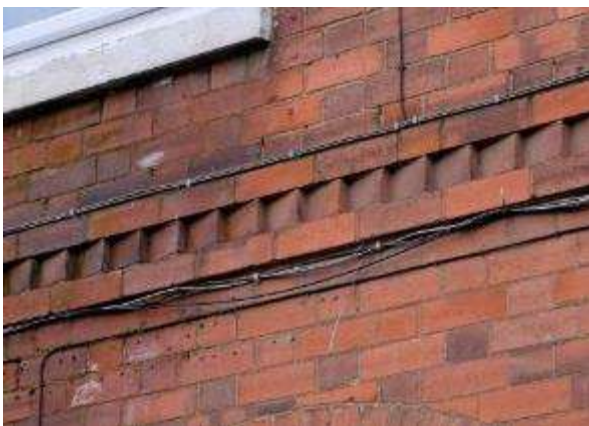
In Evesham, a corbelling course (left) and arches highlighted by contrasting brickwork in Harvington (right)
