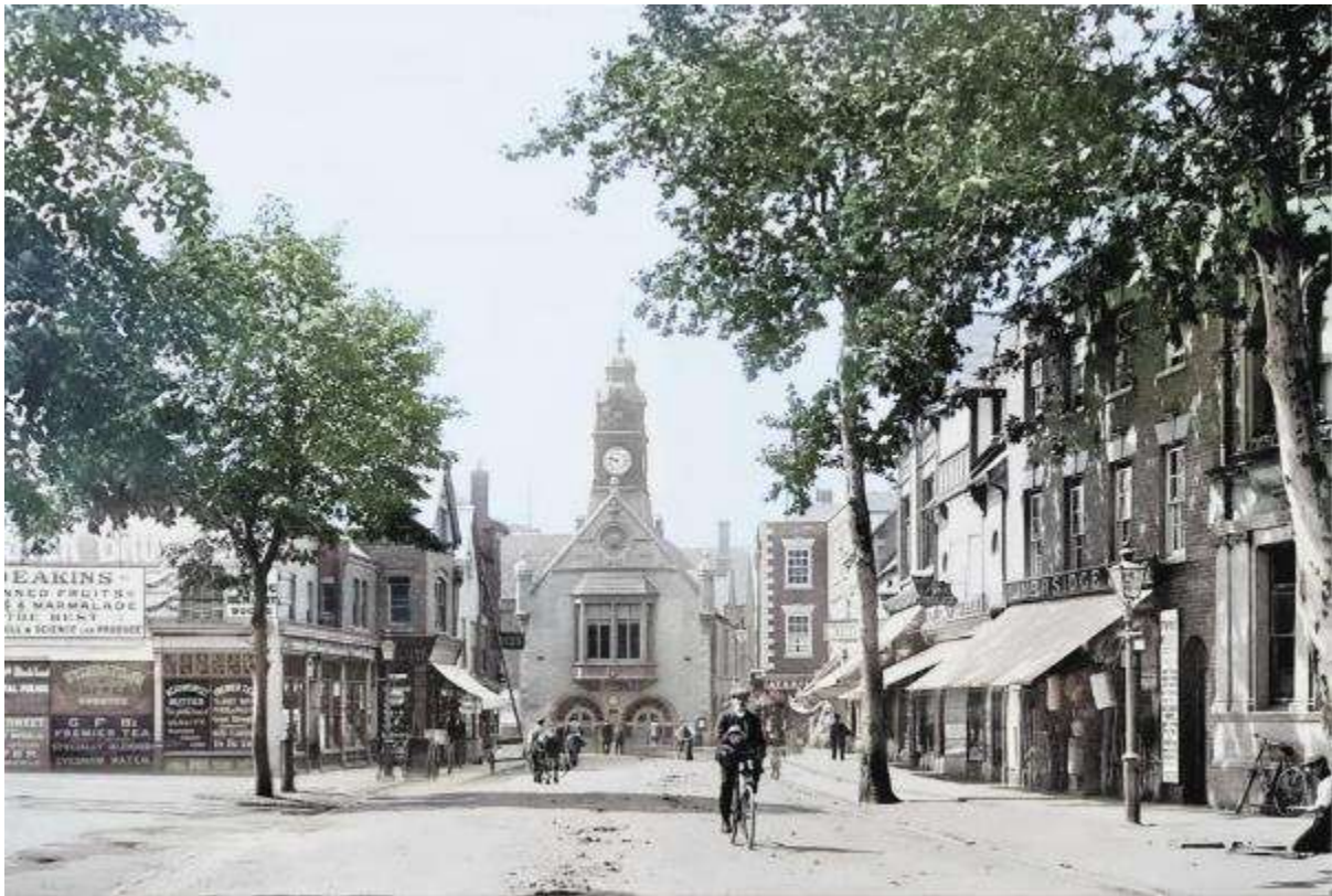
1910 photo of a tree-lined High Street in Evesham
