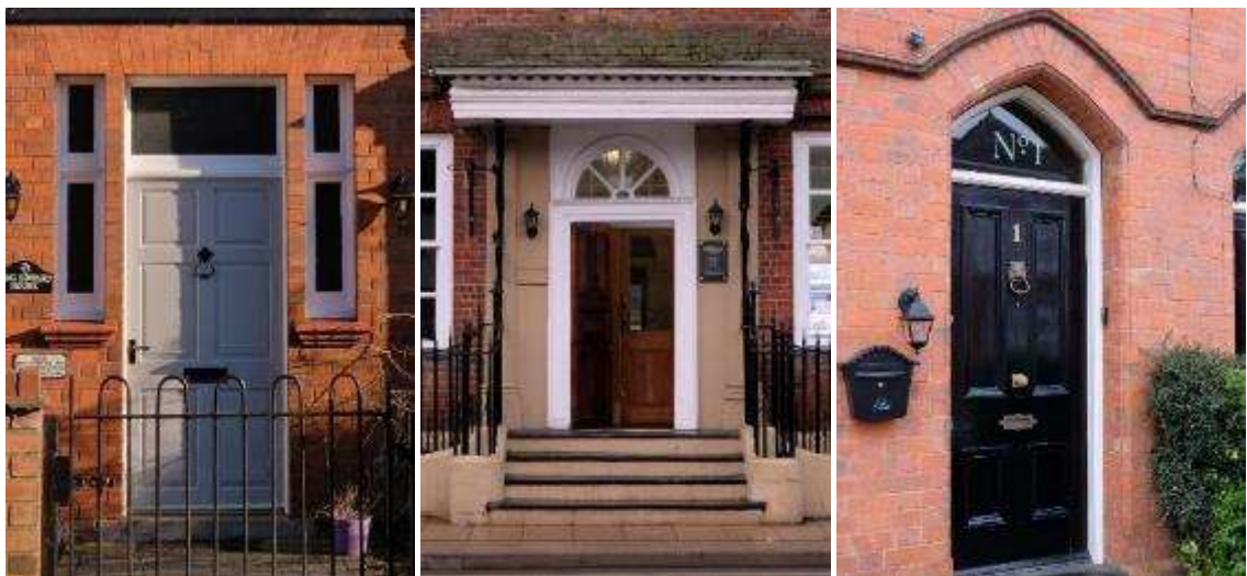
Doors in Evesham with a fanlight and small windows either side (left), a classical door with large canopy (centre) and a Gothic door (right)
