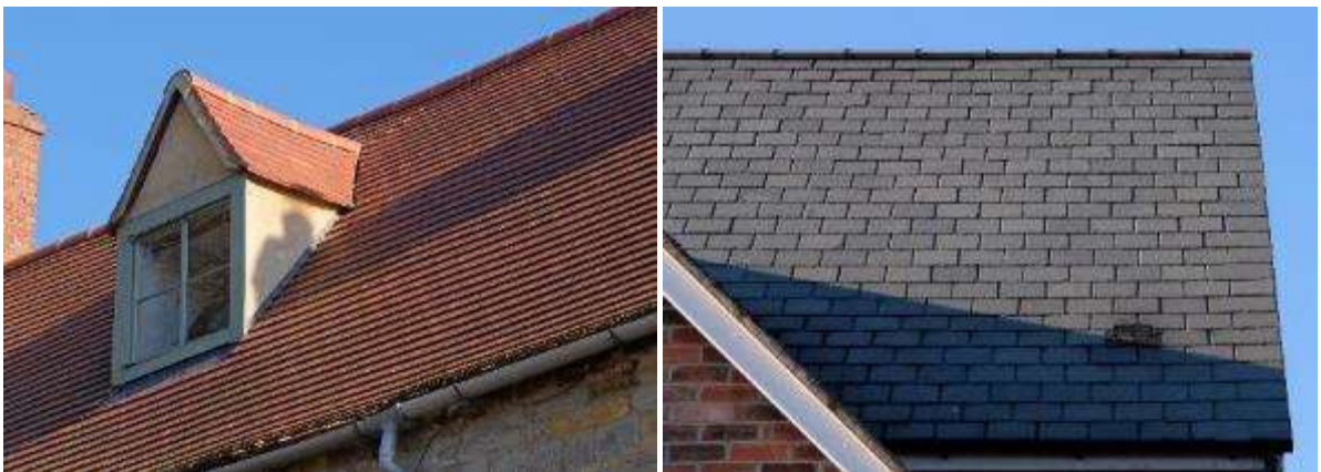
Imitation clay in Pebworth (left) and imitation slate in South Littleton (right)
