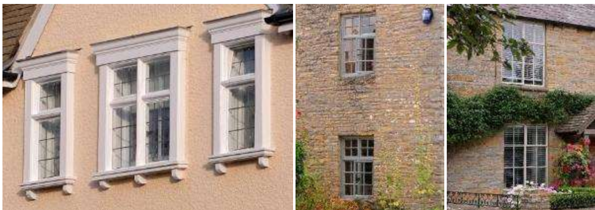
Casement windows with a mullion and transom in an Arts & Crafts home in Evesham (left) and in Bretforton (centre), and windows with a very fine frame and openable panels in Bretforton (right)
