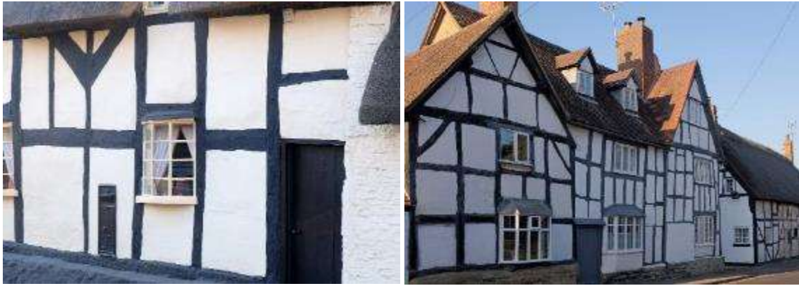
Timber framing in South Littleton (left) and Norton (right)
