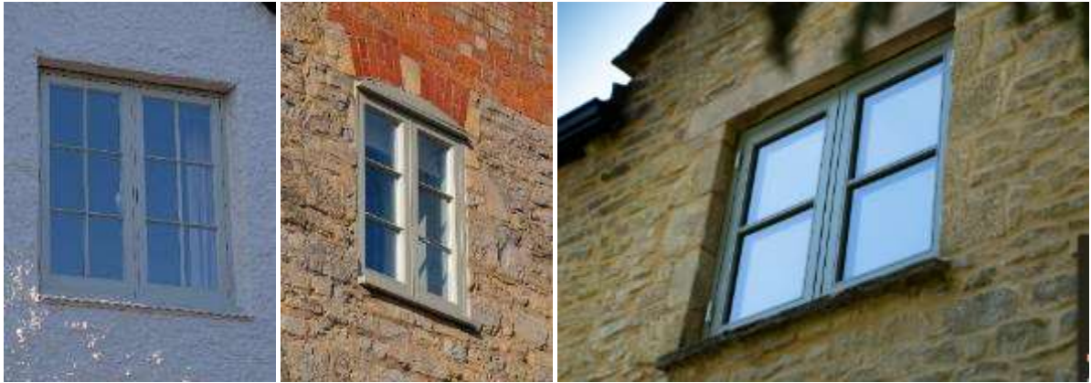
New casement windows in Pebworth (left and centre) and timber/aluminium composite casement windows (right, image credit Enlightened Windows)
