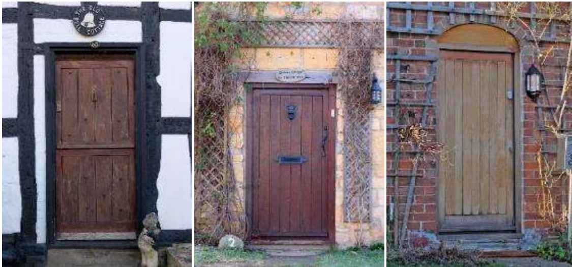
Timber panelled doors in a vernacular style in Norton (left), Honeybourne (centre) and Pebworth (right)
