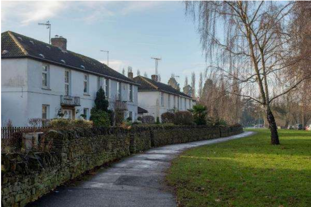
A stone front garden wall in Evesham
