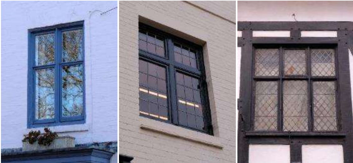
Transom casement windows in Pebworth (left), and in Evesham a multi-pane window (centre) and a diamond lattice window (right)
