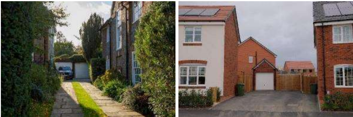
A grass strip dividing two areas of stone slabs and border planting make for a driveway (left) which is not only permeable but beautiful. Driveways which are a sea of tarmac from house to house (right) must not be built
