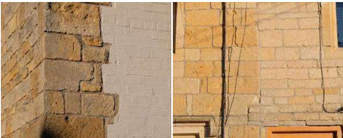
Cotswold stone alongside painted brick (left) and minor variation in tone of two Cotswold stone houses (right) in Honeybourne
