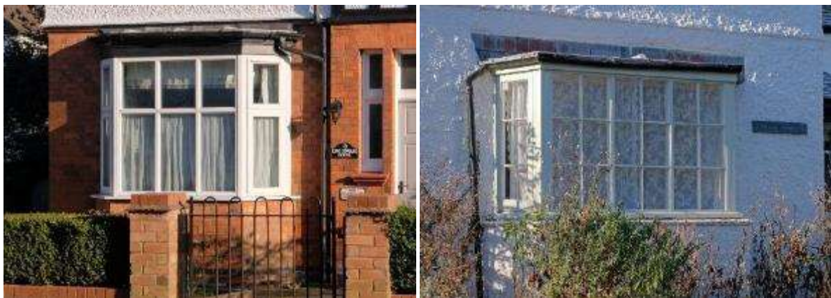
A flat-roofed bay window in South Littleton (left) and a box bay window in Pebworth (right)
