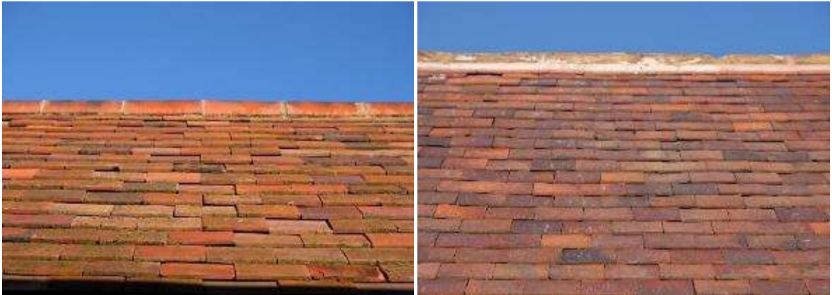
Natural clay roof tiles in Honeybourne (left) and Pebworth (right)
