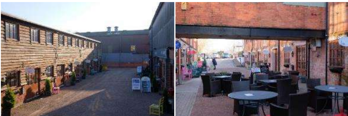
Blackminster Business Park has a number of business units of various types in a pedestrian-friendly environment appropriate for a more urban context
