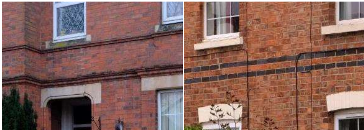
Brick string courses in Evesham (left) and a string course in contrasting brickwork in Harvington (right)
