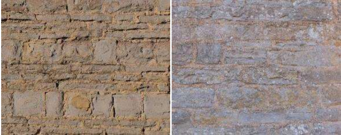
A lias stone wall in Honeybourne with alternating courses of larger and smaller stones (left) and a lias stone wall in North Littleton (right)
