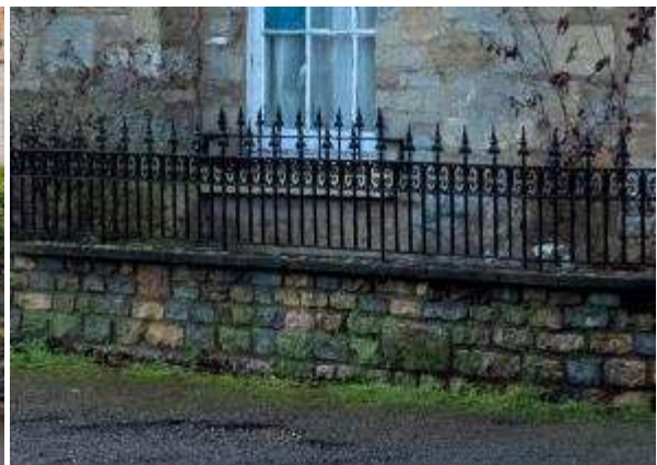
Hybrid lias stone garden walls in Evesham, with hedges (left) and iron railing (right)
