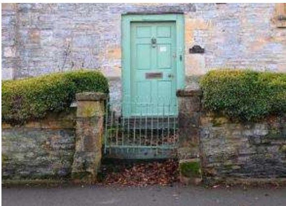
Hybrid lias stone garden walls in Evesham, with hedges (left) and iron railing (right)
