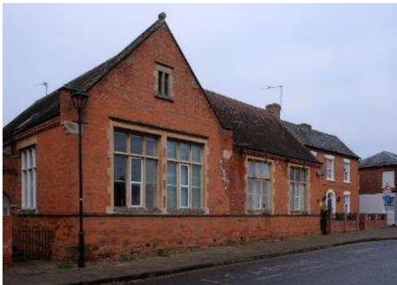
A former school building in Evesham
