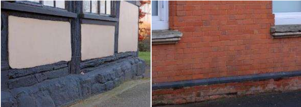
A painted stone plinth in Norton (left) and a brick plinth in Evesham (right) which shows how a plinth can take the brunt of wear and tear of a wall, helping preserve the wall above
