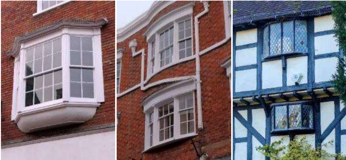
In Evesham, a single height (left) and double height (centre) oriel windows, and in Harvington two oriel windows with diamond lattice windows (right)
