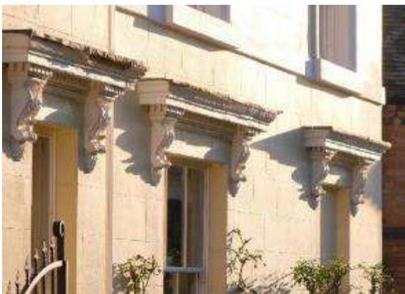
Highly ornamented window entablature in Harvington (left) and a hood mould on a Cotswold stone house in Honeybourne (right)
