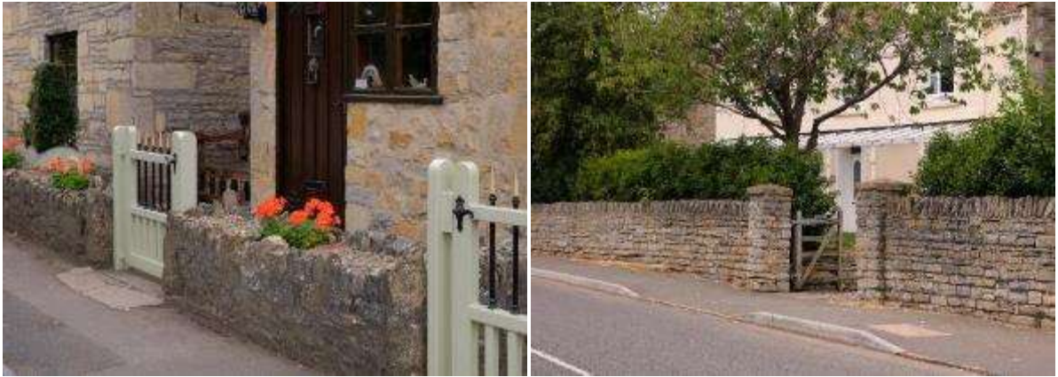
Short stone walls in Bretforton with timber gates (left) and a stone wall with hedges above in Cleeve Prior (right)
