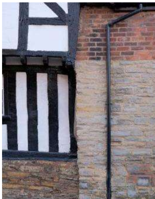
A brick, stone and timber frame wall in Harvington
