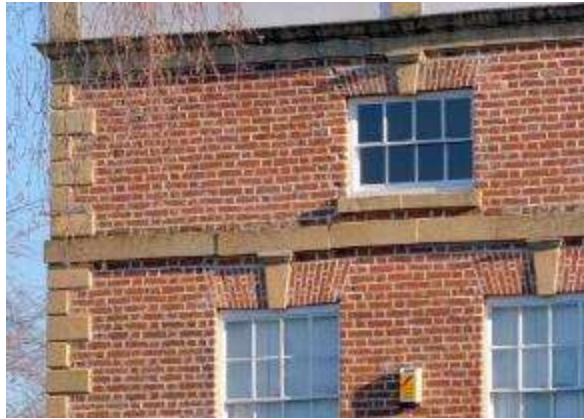
Stone quoins, a stone string course and lintel capstones in South Littleton (left) and dentils and corbels in Evesham (right)
