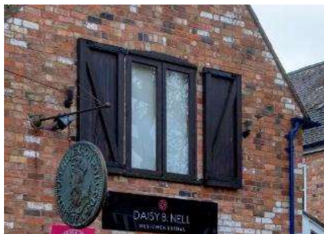
With the increased risk of overheating in recent years, shutters resembling these in Evesham can be included to control solar gain
