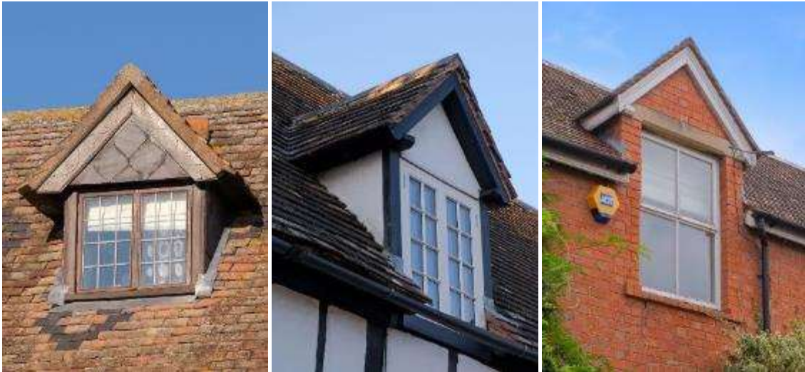
An ornated dormer in North Littleton (left) a dormer in Norton (centre) and a wall dormer in Honeybourne (right)
