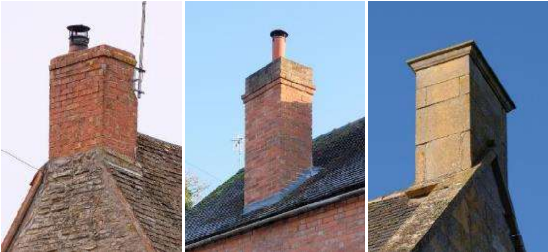
Simple yet robust brick chimneys in Bretforton (left) and Harvington (centre) and in stone in Honeybourne (right)
