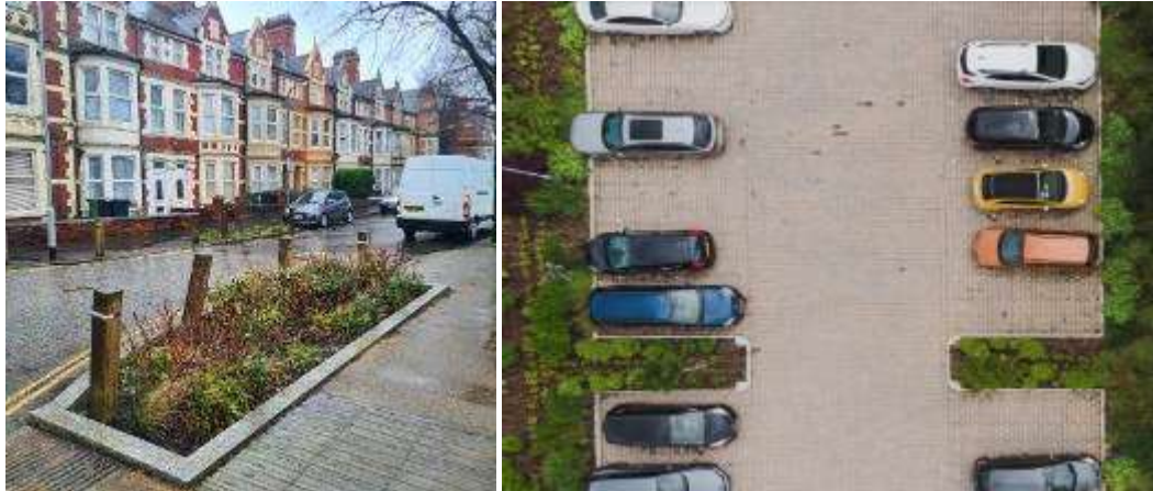
Rain gardens in Cardiff (left) are an example of SuDS appropriate for an urban development. A permeable parking area framed by SuDS creates a pleasant environment for a business unit in Evesham (right, image credit Susdrain)
