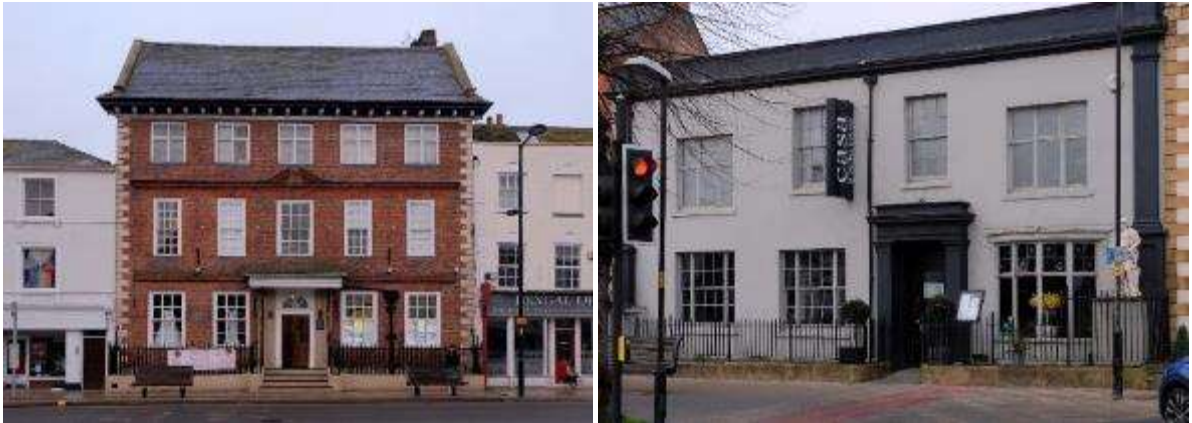
Commercial and mixed-use buildings in Evesham
