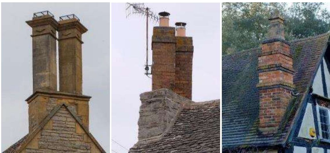
Dual chimneys in Bretforton (left) and Cleeve Prior (centre) and a substantial chimney with bands of darker bricks in Harvington (right)
