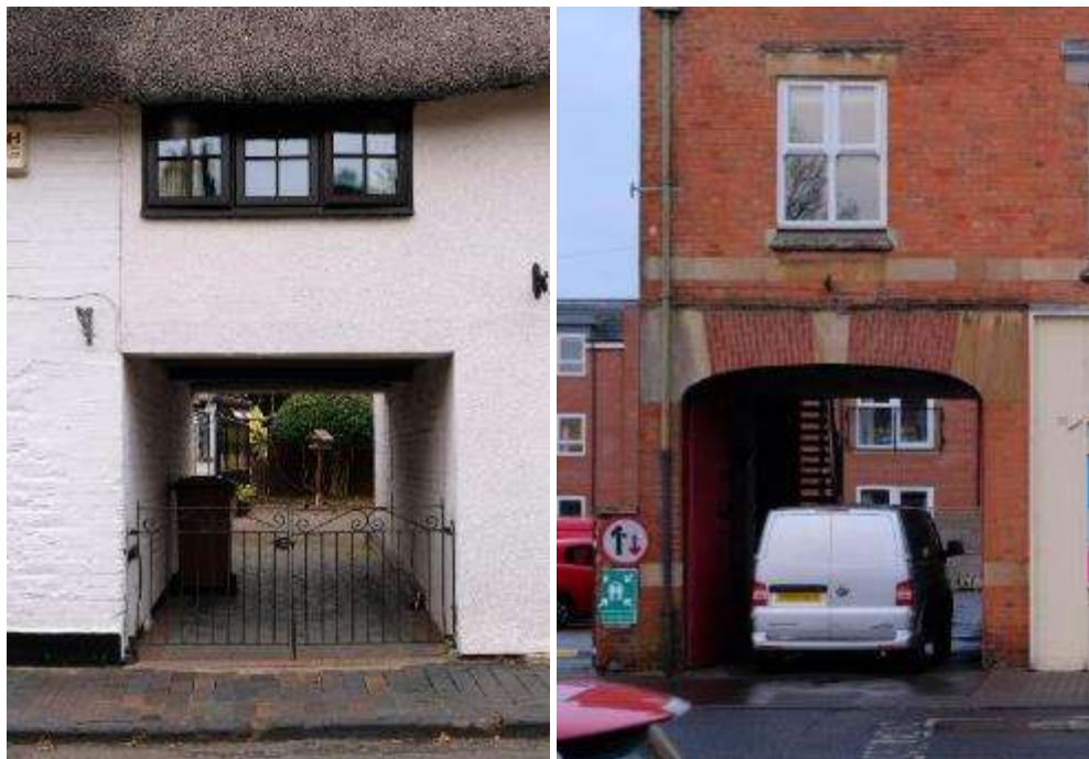
Covered passageways as here in Bretforton (left) and Evesham (right), with or without gates or doors, can help preserve a building line and provide additional floor space above
