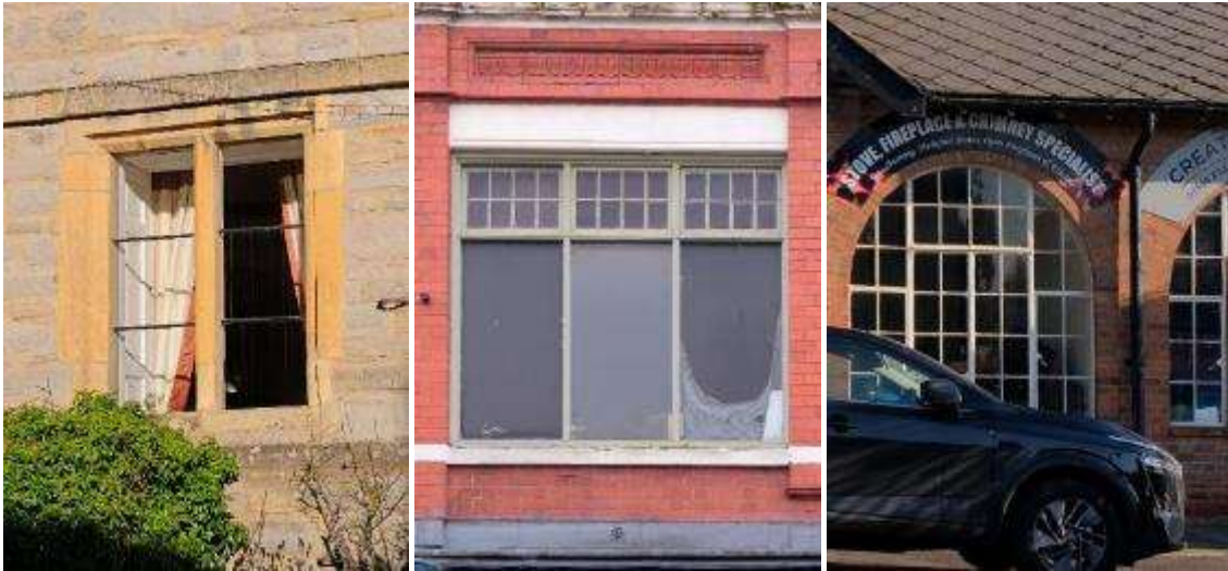
Fixed windows in Pebworth (left), windows with a transom and top hung fanlights in Evesham (centre) and arched multi-pane windows in Blackminster (right)
