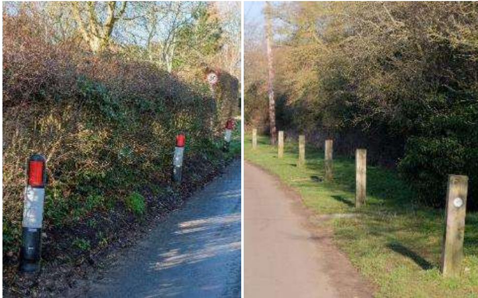
Plastic bollards must not be used (left). Instead, in villages and rural areas, timber bollards are a more sympathetic option, such as these in South Littleton (right)
