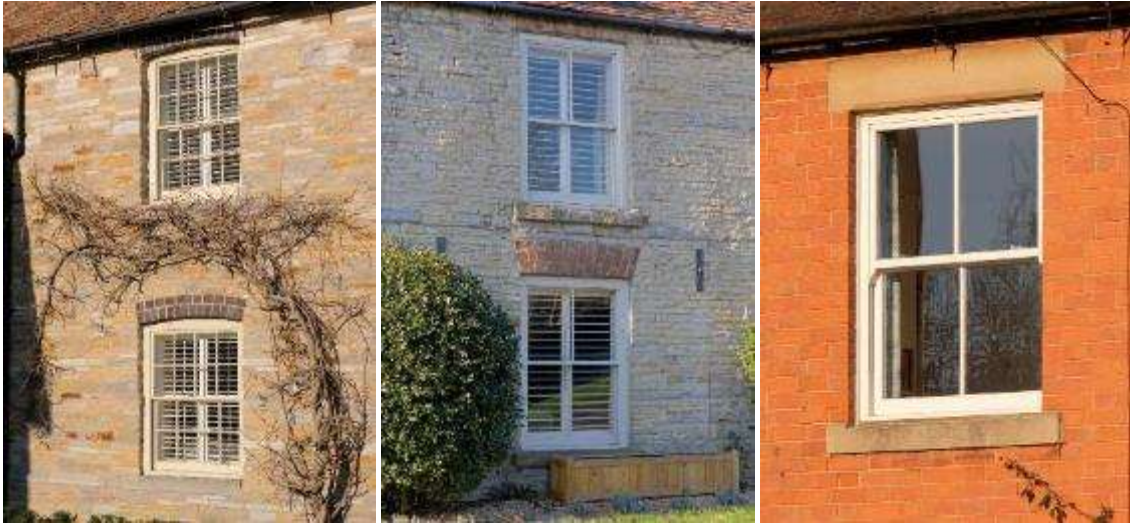
8-over-8 and 2-over-2 sash windows in North Littleton (left and centre), and 2-over-2 sash windows in Harvington (right)
