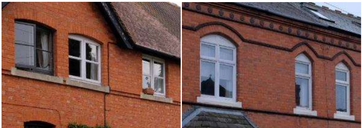
2 pane casement windows in Bretforton (left) and casement windows with a transom in Evesham (right)
