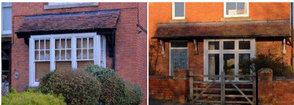
Box bay windows in Evesham (left) and in combination with a door canopy in Harvington (right)
