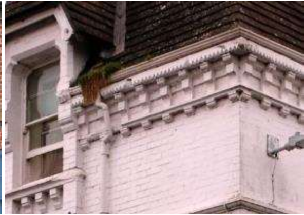
Stone quoins, a stone string course and lintel capstones in South Littleton (left) and dentils and corbels in Evesham (right)
