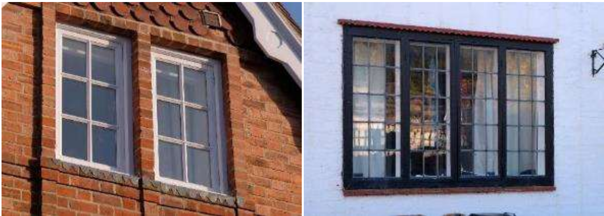
Dual casement windows in Evesham (left) and a window with mullions in South Littleton (right)
