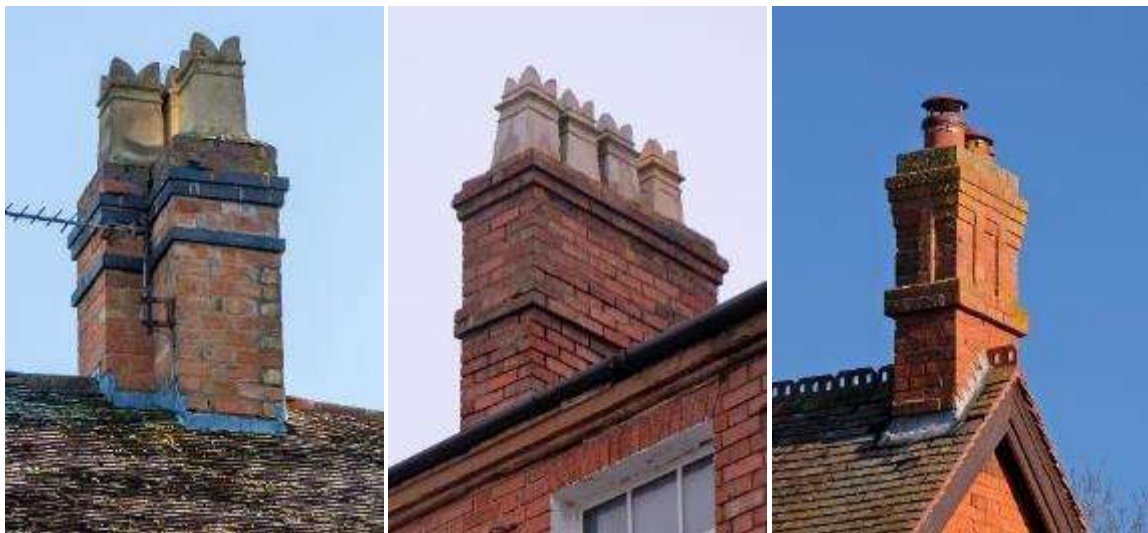
Chimneys with square pots in Pebworth (left) and Evesham (centre) and a chimney with complex brickwork in Honeybourne (right)
