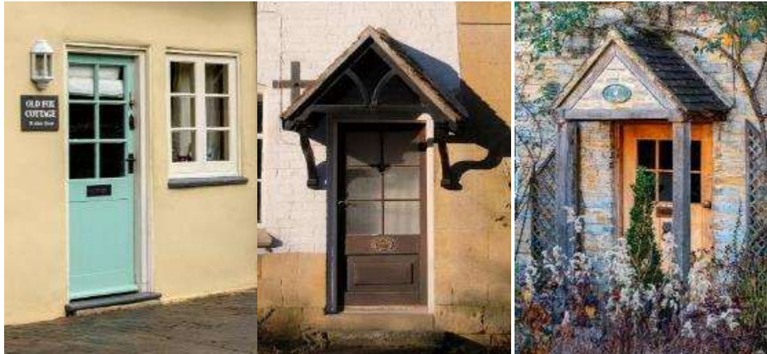
Timber panelled doors in a vernacular style and with glazing in Bretforton (left), and in Honeybourne (centre) and Pebworth (right) with simple pitched timber canopies
