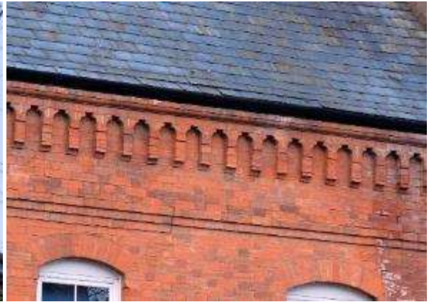
In Evesham, dentilled eaves corbels (left) and an elaborate brick frieze (right)
