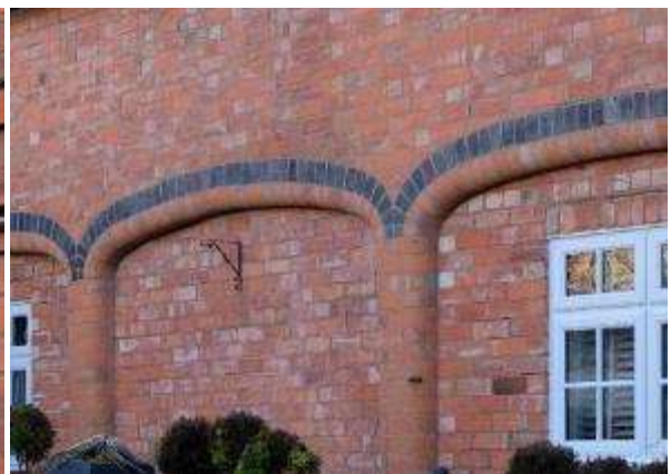
In Evesham, a corbelling course (left) and arches highlighted by contrasting brickwork in Harvington (right)
