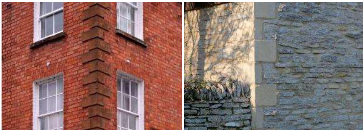
Stone quoins on a brick building in Evesham (left) and on a lias stone house in North Littleton (right)
