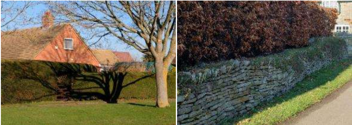
Hedge boundary in Honeybourne (left) and combination stone and hedge boundary in North Littleton (right)
