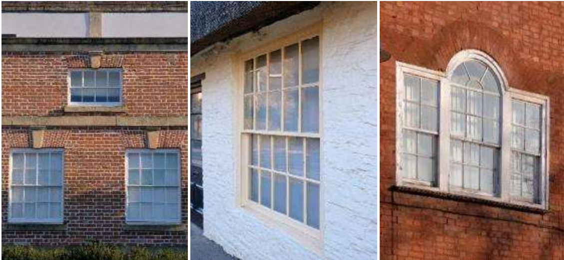
4-over-4 sash windows (left) and 10-over-10 sash windows (centre) in South Littleton and in Evesham a unique Venetian sash window (right)
