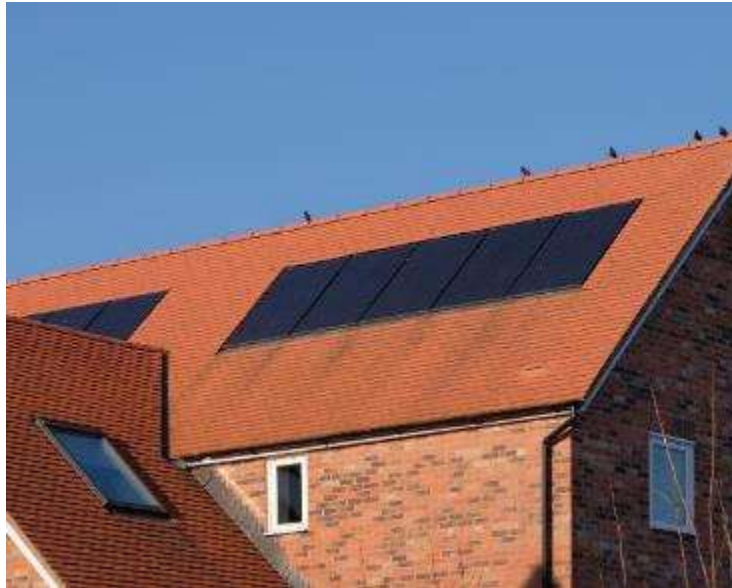
Solar panels integrated flush with the roof on a house in South Littleton
