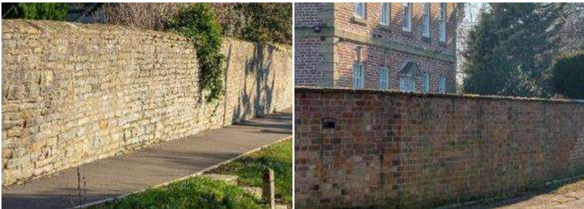
Lias stone boundary wall in Pebworth (left) and a brick boundary in South Littleton (right)
