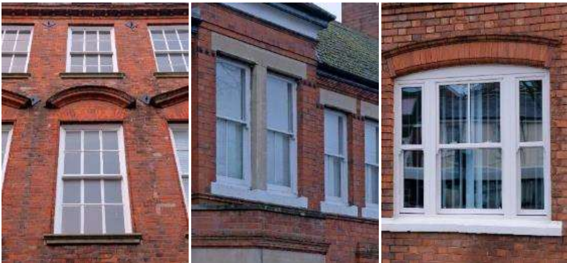
Large 6-over-6 sash windows (left), 1-over-2 windows (centre) and coupled 1-over-1 and 2-over-1 windows (right) in Evesham
