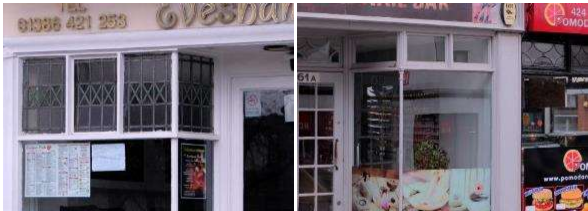
Detailing such as on these shopfronts in Evesham should be preserved where it still exists and restored where possible
