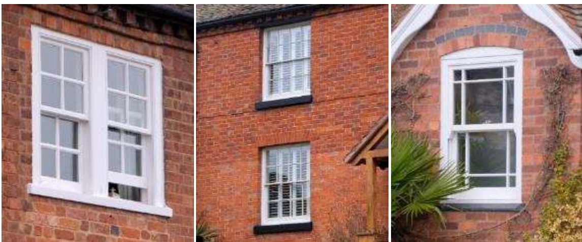
A pair of 4-over-4 sash windows in Crothorne (left), and in Crowle 8-over-8 sash windows and a unique 6-over-6 sash window (centre and right)
