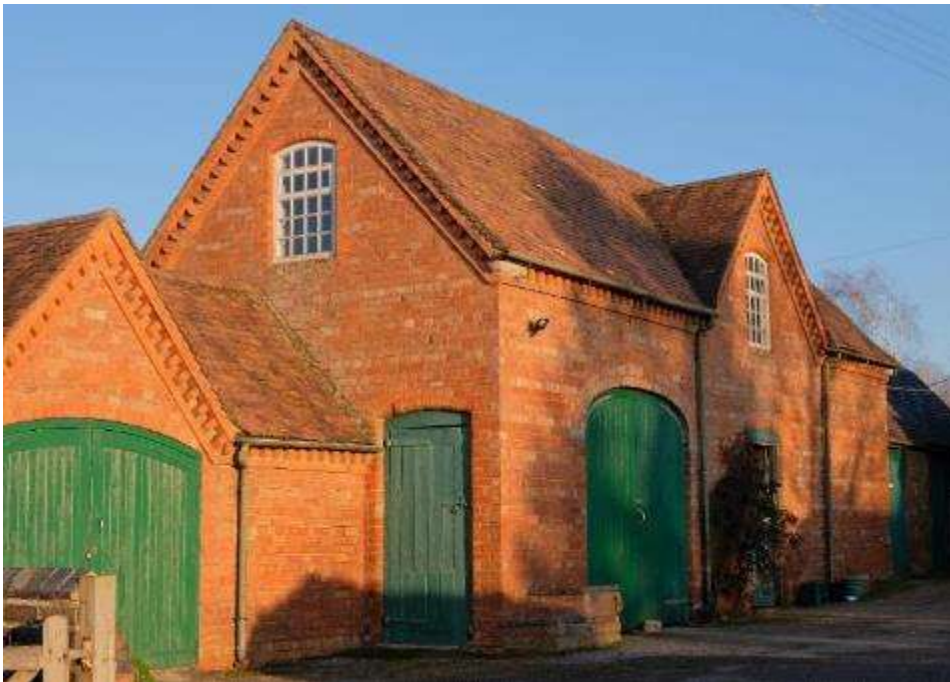
This building in Atch Lench can be a model for a mews house with its large doors and living space above
