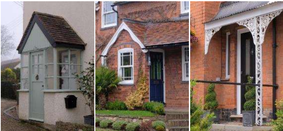
Enclosed porches in Eckington (left) and Crowle (centre) and an iron porch in Persore (right)
