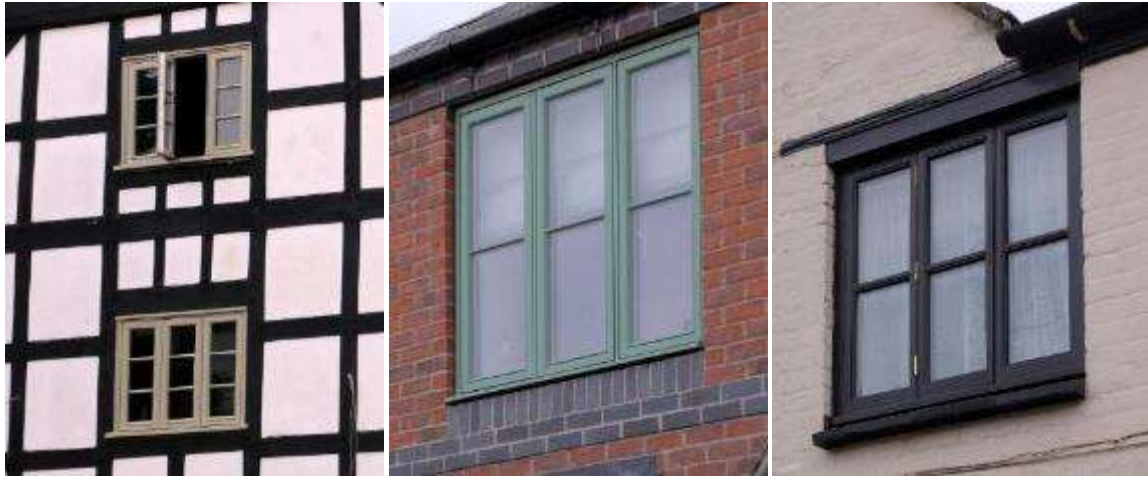
2 and 3 pane casement windows in Bishampton (left), Crowle (centre) and Eckington (right)
