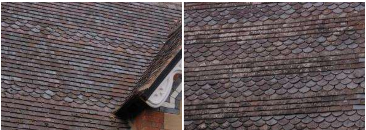
Roof tiles with bull nosed bands in Rous Lench (left) and Wick (right)
