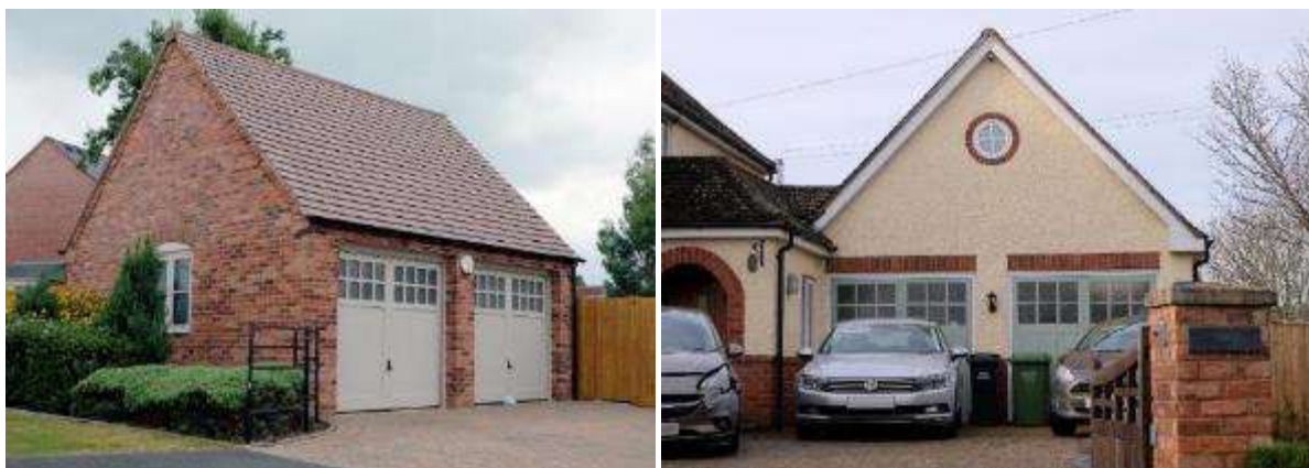
A new-build brick garage in Crowle (left) and a rendered garage in Great Comberton (right)
