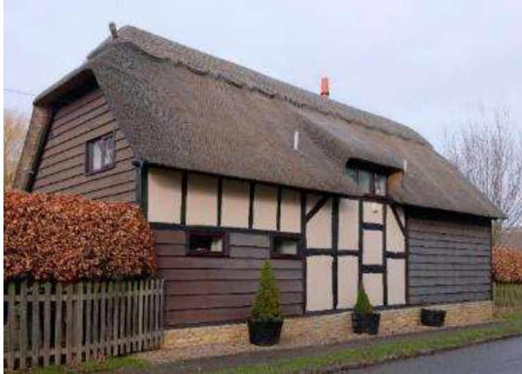
A primarily timber-clad house in Great Comberton
