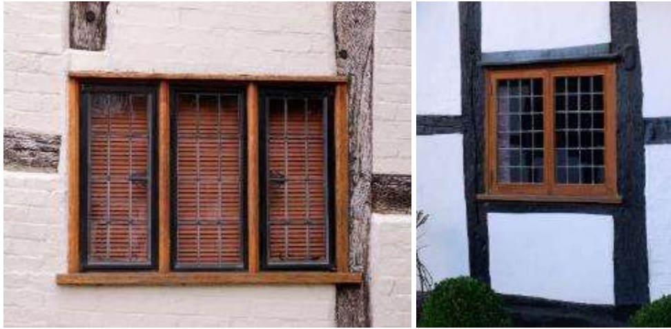
Square leaded steel windows within a timber frame in Crowle (left) and wholly timber in Little Comberton (right)
