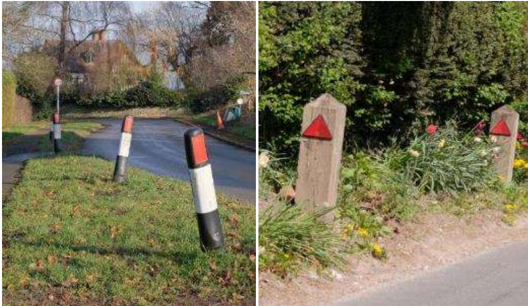
Plastic bollards must not be used (left). Instead, in villages and rural areas, timber bollards are a more sympathetic option (right)
