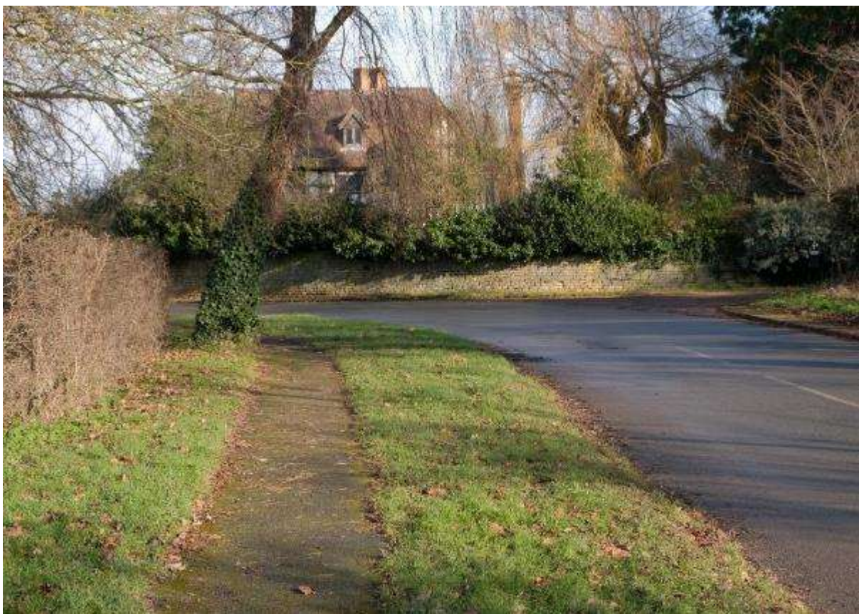
On streets without kerbs, such as this street in Little Comberton, verges can play an important role in absorbing street runoff
