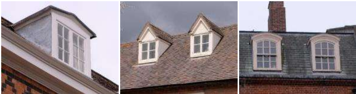
Dormer windows in Fladbury (left) and Persore (centre) and dormers within a mansard roof in Persore (right)
