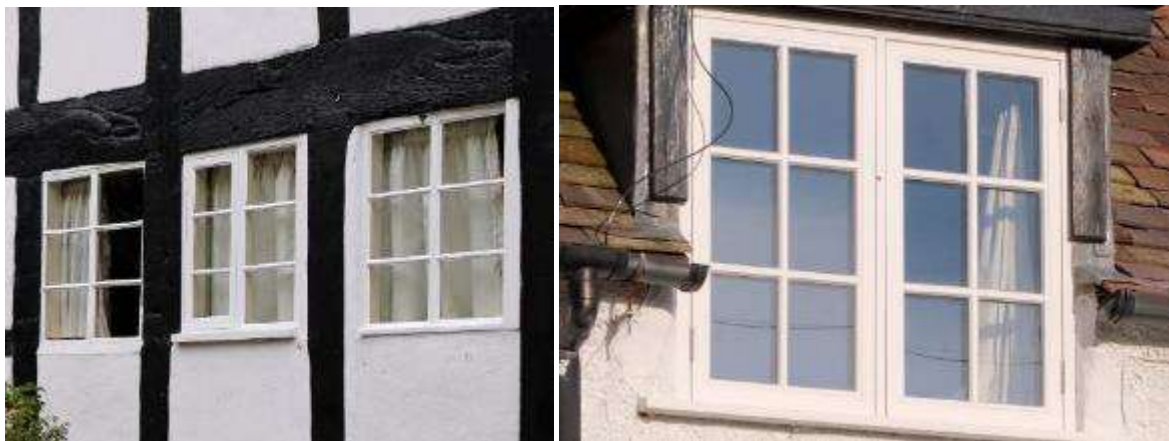
A group of casement windows in Crophorne (left) and a 6 panel casement windows in Great Comberton (right)
