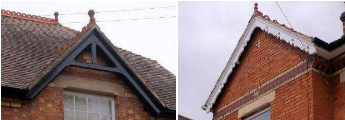
Ornamental bargeboards and finials atop gables in Fladbury (left) and Pershore (right)
