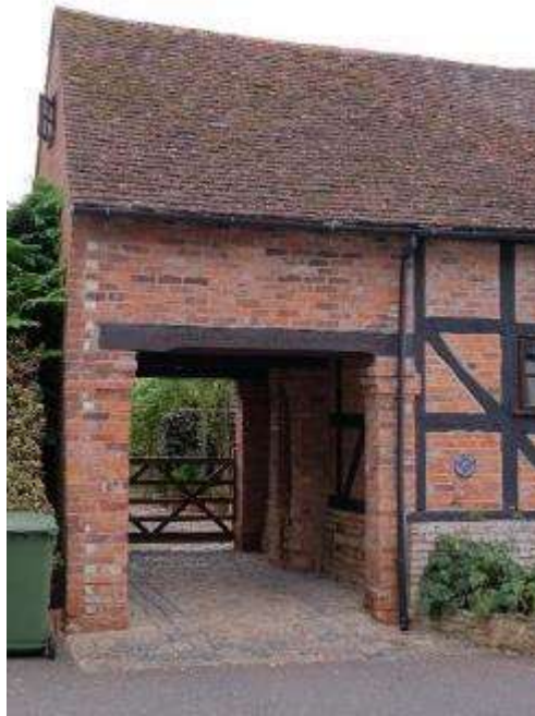
In a village setting, a covered passageway in Crothorne leads to a driveway and garage behind
