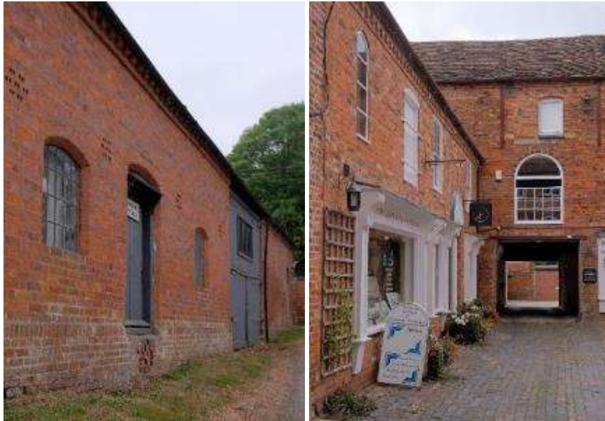
A small industrial building in Crophorne (left) can serve as a model for a commercial or workshop space, and retail buildings in Pershore (left)
