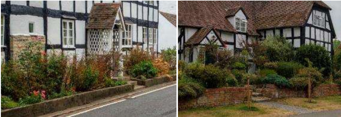
A short stone wall with planting in Crophorne (left) and in Bishampton (right) a brick wall with a generous setback from the street
