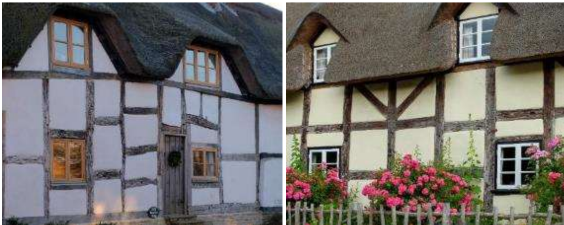
Houses with unpainted timber frames in Atch Lench (left) and Crowle (right)
