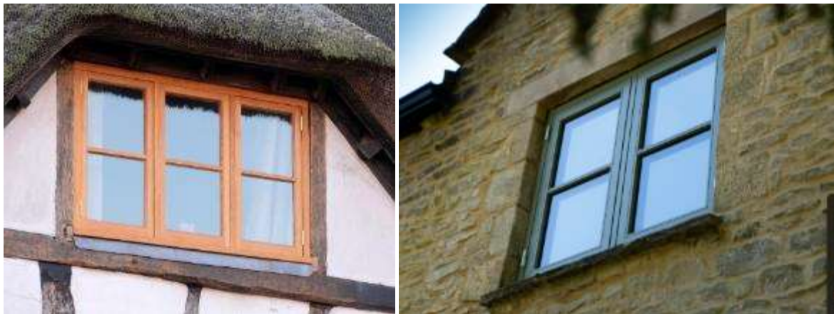
Casement windows on a house in Atch Lench (left) and timber/aluminium composite casement windows (right, image credit Enlightened Windows)
