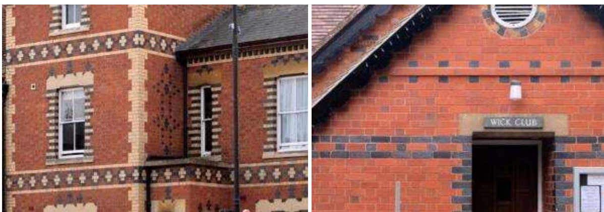
Contrasting brickwork, including string courses, quoins and window surrounds, on a house in Persore (left) and on the village club in Wick (right)
