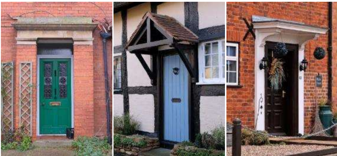
A brick porch in Eckington (left), a timber porch in Little Comberton (centre) and a classical porch in Crophorne (right)
