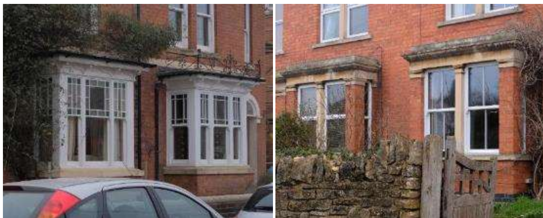
Pairs of large Victorian bay windows in Eckington in brick and timber (left) and brick (right)
