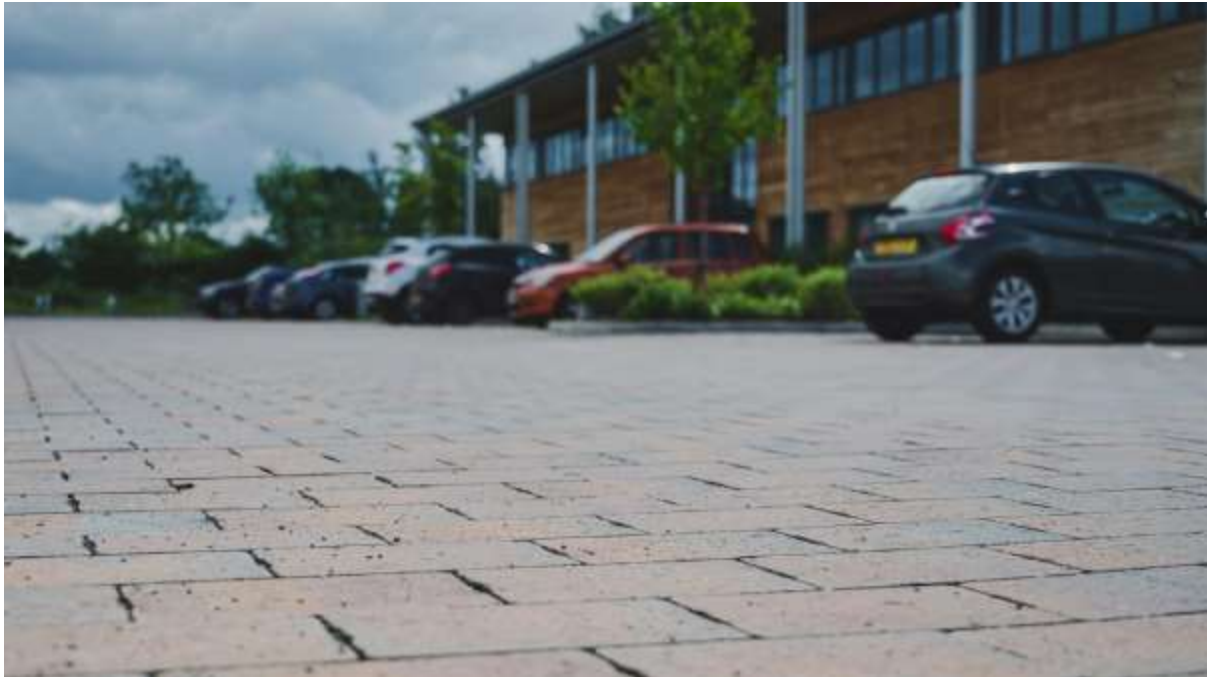
Permeable brick paving at the Robert Welch facility in Evesham (Image credit Susdrain)
