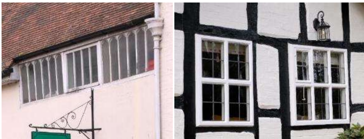
Wide horizontal windows in Persore (left) and fixed windows with a small openable panel in Great Comberton (right)
