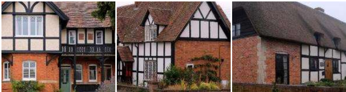
Hybrid timber frame homes with partially brick walls in Wick (left), Church Lench (centre) and Eckington (right)
