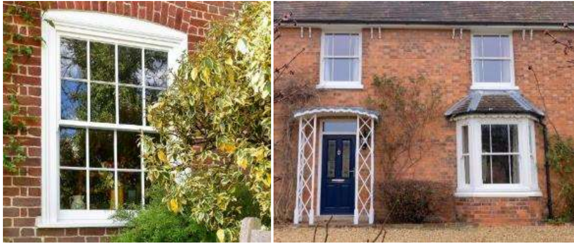
New sash windows (left, image credit Timber Windows) and 3-over-3 sash windows on a house in Eckington (right)
