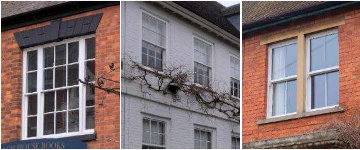
Coupled 6-over-6 and 2-over-2 sash windows in Pershore (left), and 6-over-6 sash windows and a pair of 2-over-2 sash windows (right) in Eckington
