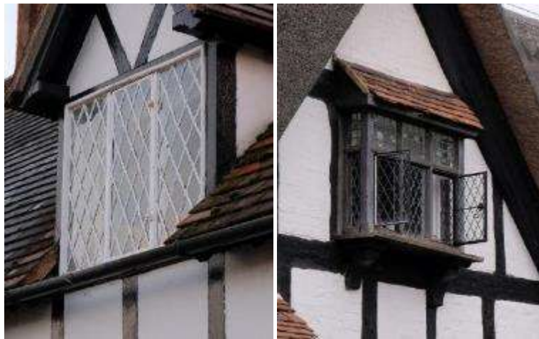
Diamond paned windows in Church Lench (left) and within an oriel window in Crophorne (right)
