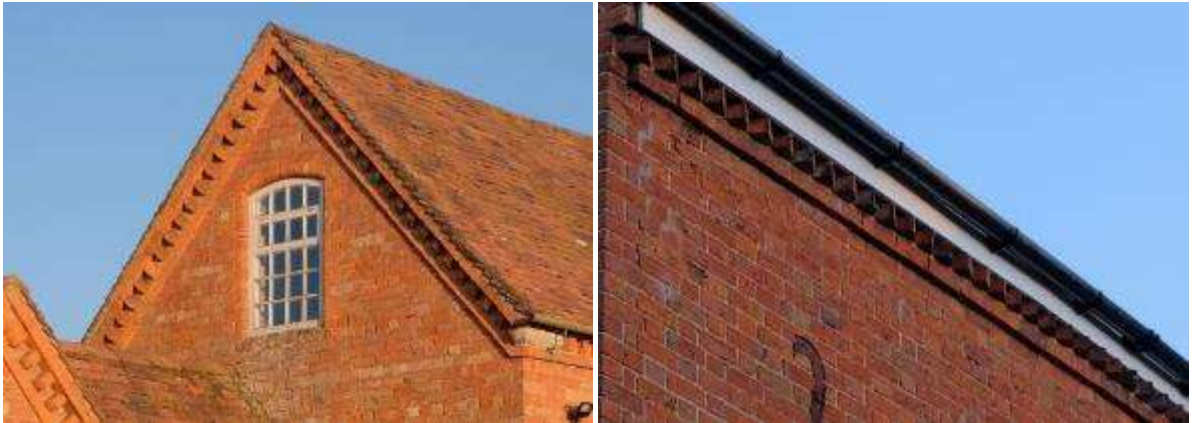
Dentilled eaves corbels in Atch Lench (left) and a dogtooth dentilled eaves course in Fladbury (right)
