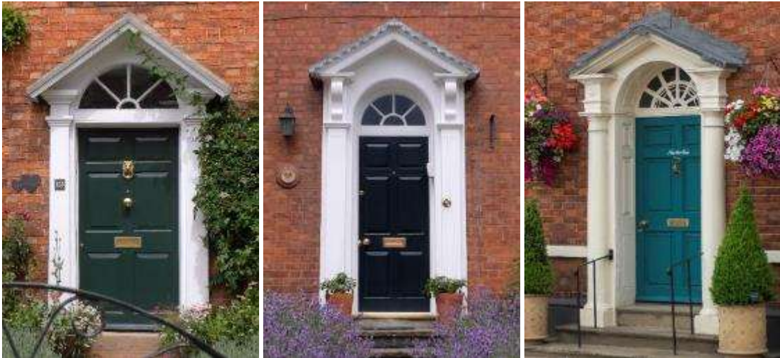
A classical door and door canopy or porch can be an appropriate choice for a formal, classically designed house, such as these Persore examples
