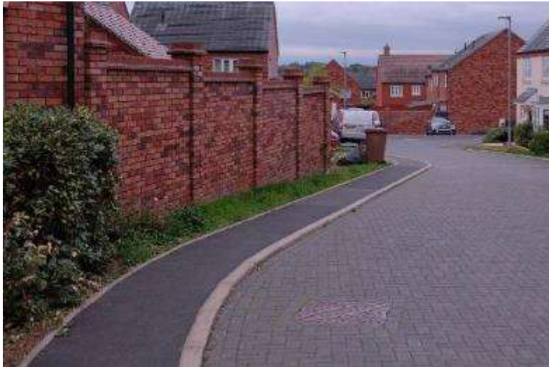
Pavements barely wide enough to walk along, such as this example in Persore, will no longer be acceptable
