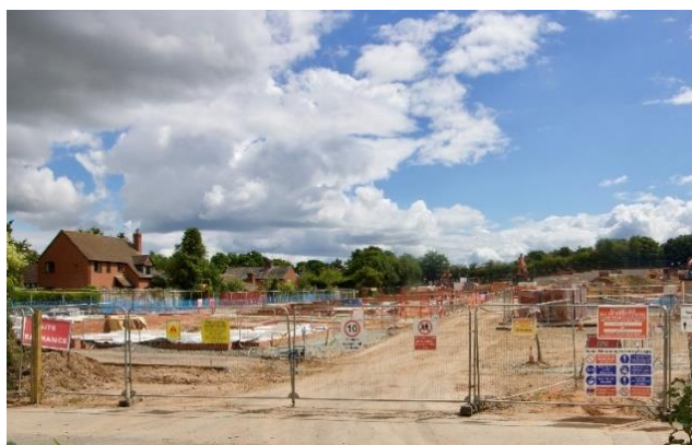
'The Racks' development being built
