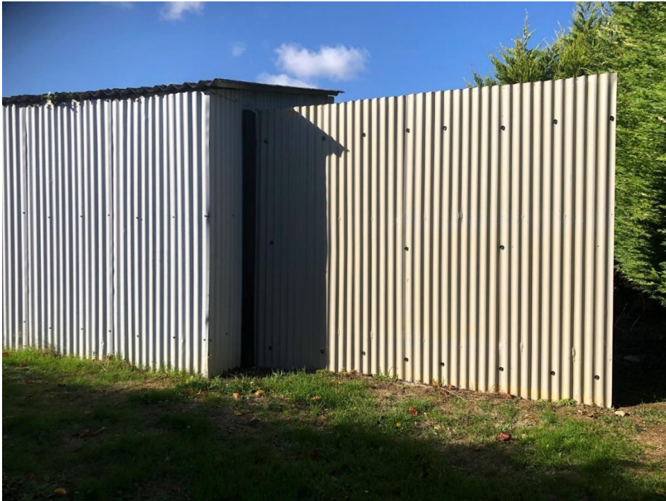
Figure 4 – GS3 Land to rear of Church on 10/10/2022
