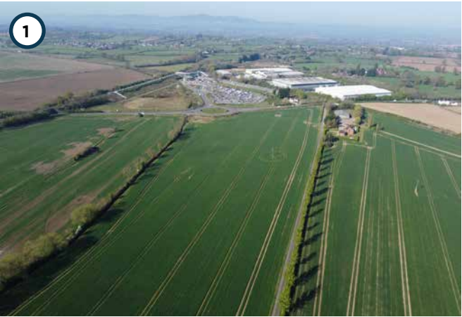
The existing station is approached by a ridge, that sits between two valleys (left and right of image).
