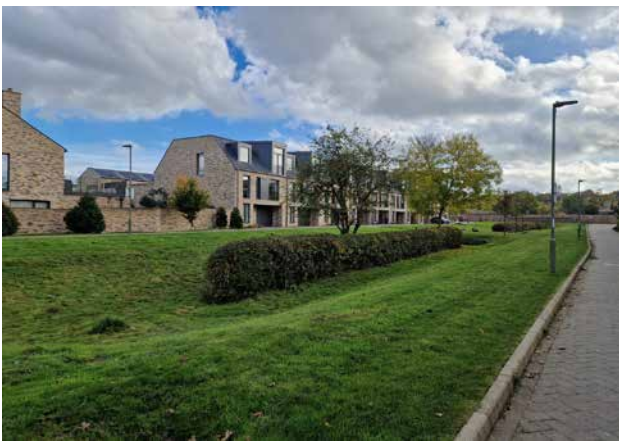
Swales and water management integrated with streets
