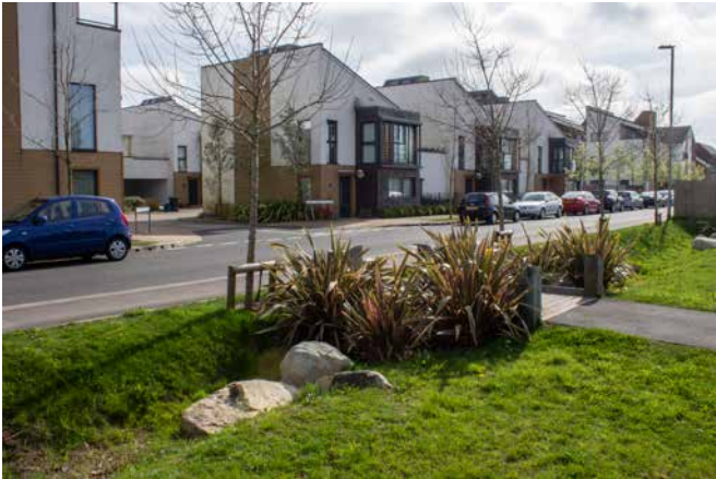
Planted street swales for infiltration or conveyance
