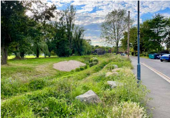
Check dams within swales to slow flow and provide permanent water
